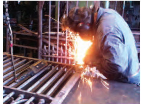
Blacksmith repairing wrought iron graveyard gates in West Cork.
