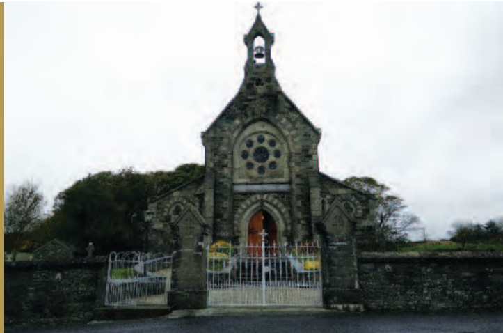
RC Church of the Most Holy Rosary, Kilcoe, dated 1905, with typical side aisles. Image courtesy of Paul Power.
