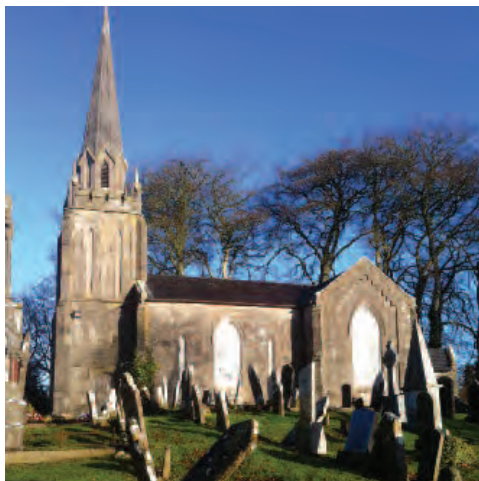
The Church of Ireland church in Castletownroche was built in 1825 and is a handsome structure built on a prominent location on the site of an earlier church. The west tower is surmounted by a finely proportioned octagonal spire. Its construction was aided with a loan of £1250 from the Board of First Fruits.
