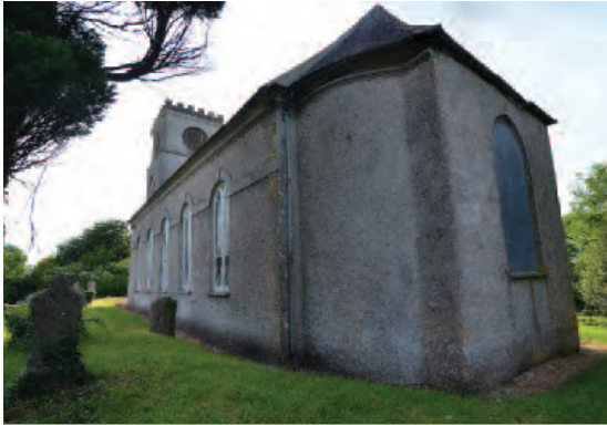
The church from south east showing the apse and the interesting band course uniting the five window in the south wall.
