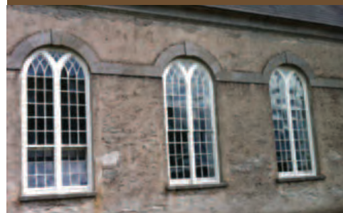
Detail of timber Y - tracery windows with delicate switch line tracery and original glass with curved cut stone cornice under eaves.
