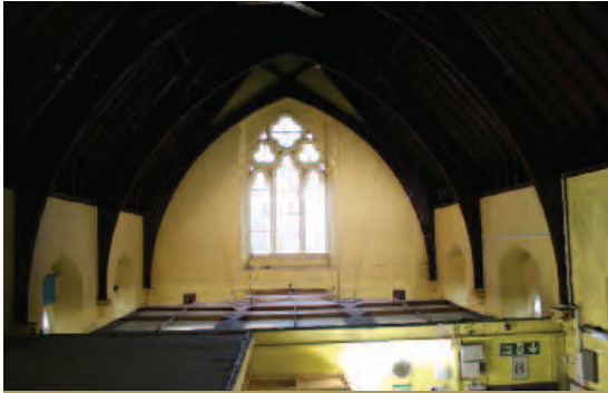
Interior showing west tracery window and fine open timber roof supported on corbels
