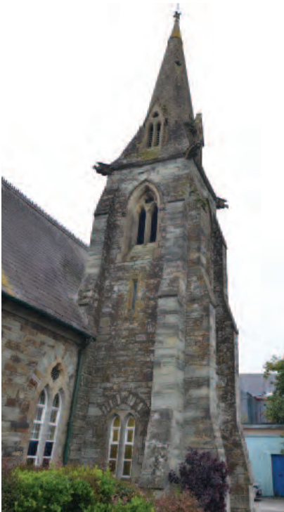
Bell tower with corner buttresses and projecting gargoyle like eagles.
