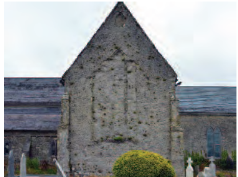
Exterior view of South Transept, showing blocked 13th century windows.
