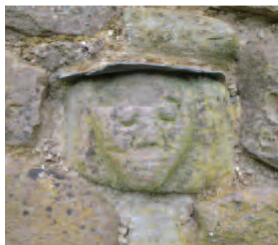
Carved stone head inserted over the door in the south wall.
