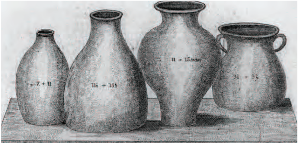
Sketch by Edward Fitzgerald of the acoustic pots found in the chancel walls during 19th century renovations.
