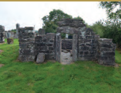
BELOW: Church at Labbamologa with trabeated doorway at west end.
