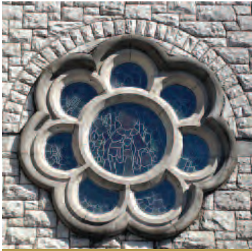
Neo-Gothic Style Oculus Window surrounded by rusticated stone work Holy Rosary Midelton.
