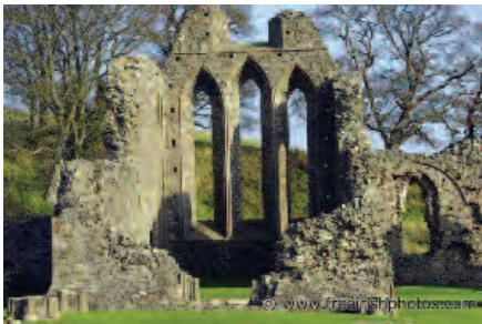
Lancet windows at Inch Abbey.
