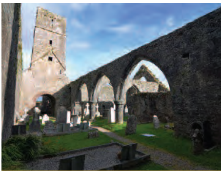
Nave of church, pointed arcading opening to the southern aisle.
