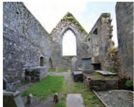
Chancel of church looking east.
