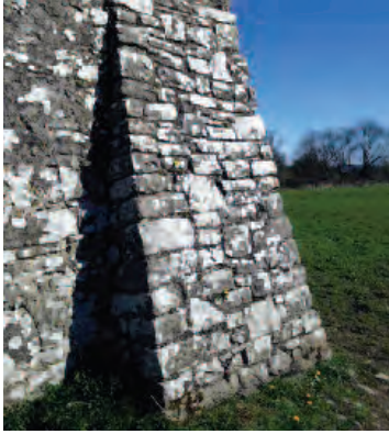
LEFT: Buttress at Ballybeg Abbey, Buttevant.
