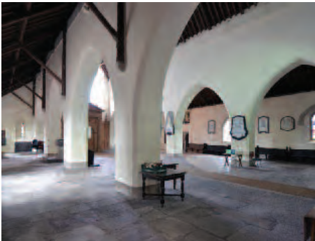
View of Nave from southeast corner of side aisle.
