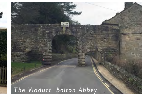
The Viaduct, Bolton Abbey
