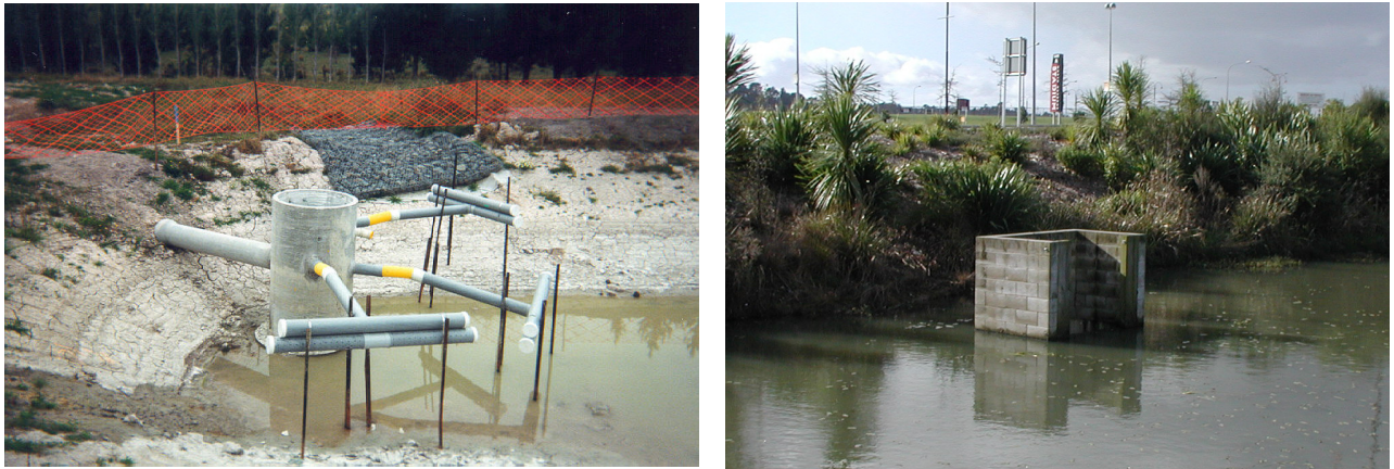
Figure 3.6. Sedimentation Basin Outlet Structures (L) a floating skimmer and (R) a narrow weir
