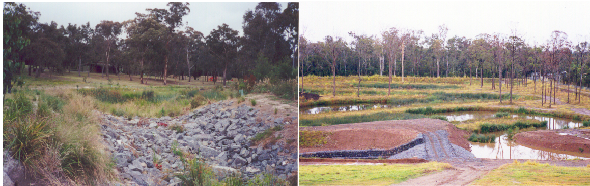
Figure 3.8. Overflow Structure of a Sedimentation Basin
