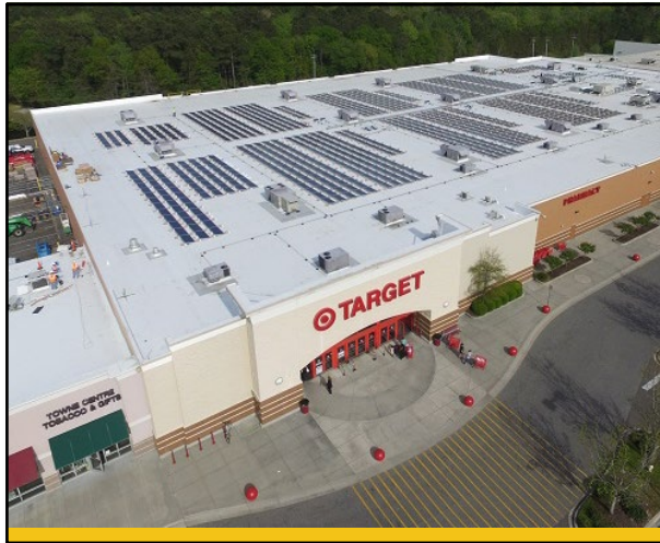
Hannah Solar North Charleston Site.
