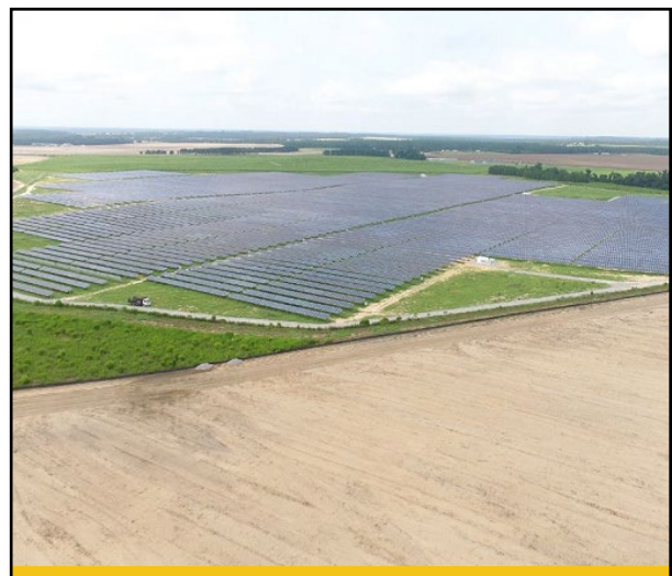
Pine Gate Renewables Odyssey Solar Farm.
