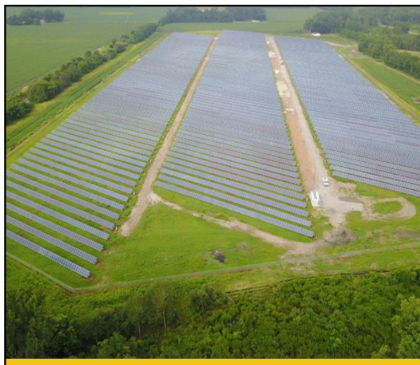
Pine Gates Renewables Cameron Solar Farm.
