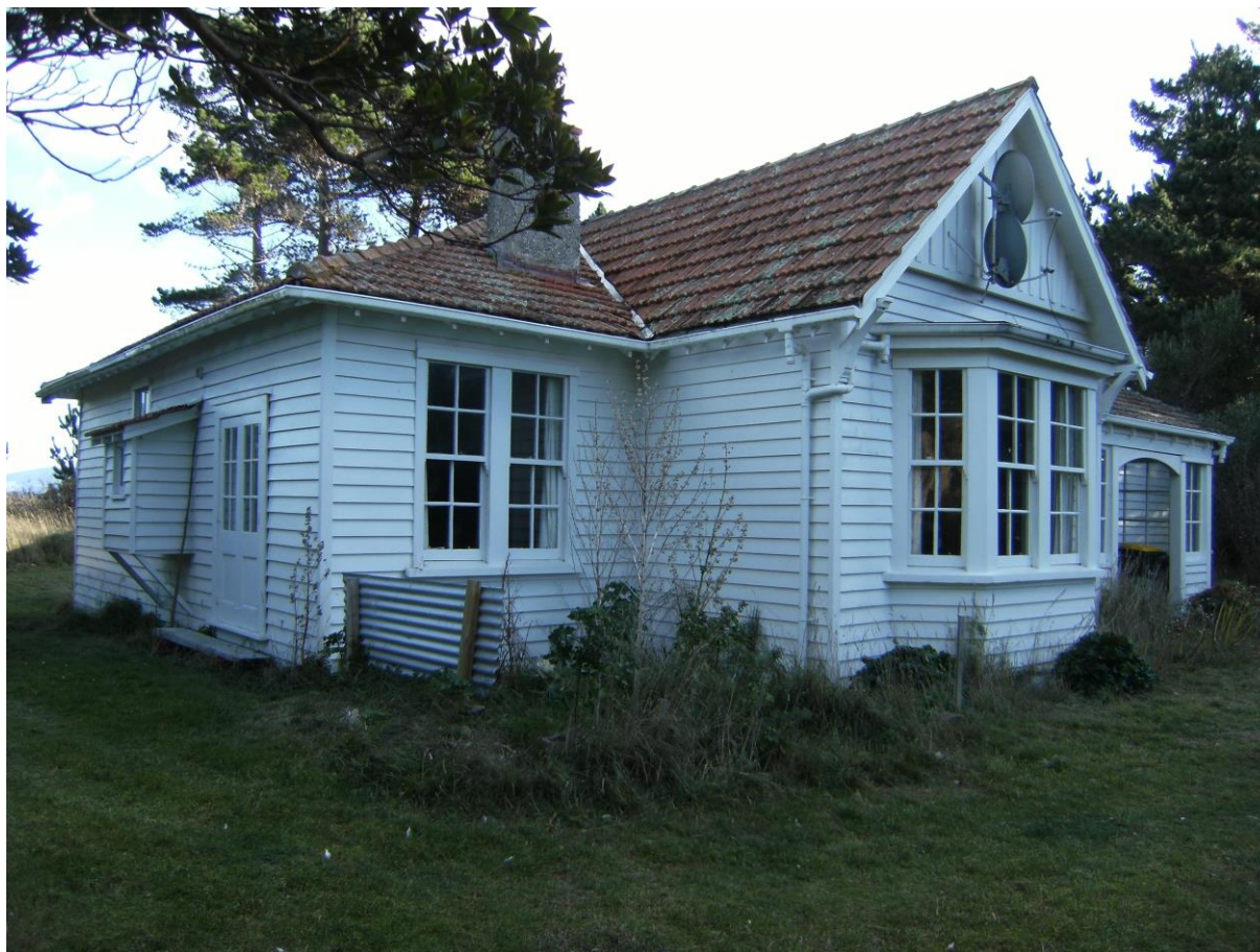
Figure 1: Cottage/pilot house No. 1 photo (July 2015)
