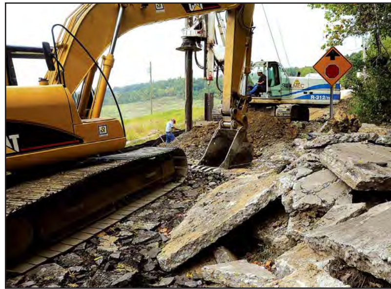
Workers tear up damaged concrete on River Road.
