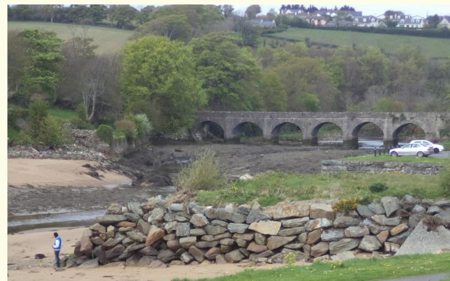
Castle Bridge, Buncrana shore front, May 2014.
