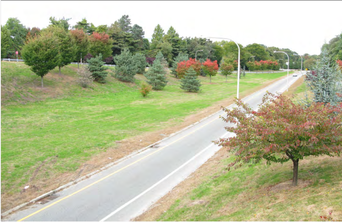
The RI Route 10 exit ramp. Vehicle speeds decrease as motorists approach the intersection with Park Ave.
