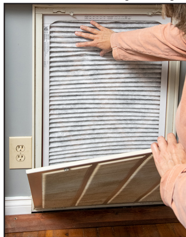
Improve your HVAC system's efficiency by checking the filter regularly and replacing it when dirty.
