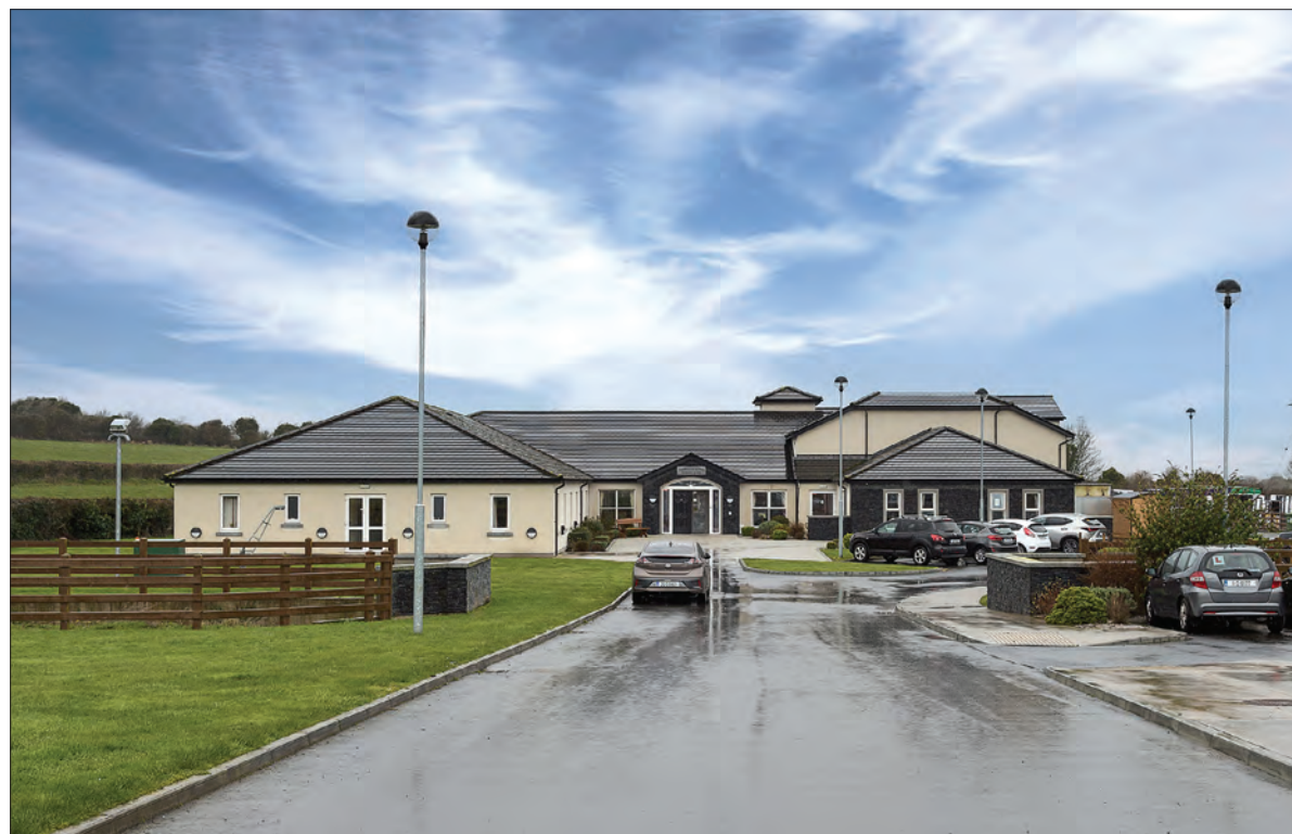
DEVELOPMENT: Millbrook Manor Nursing home in Saggart
