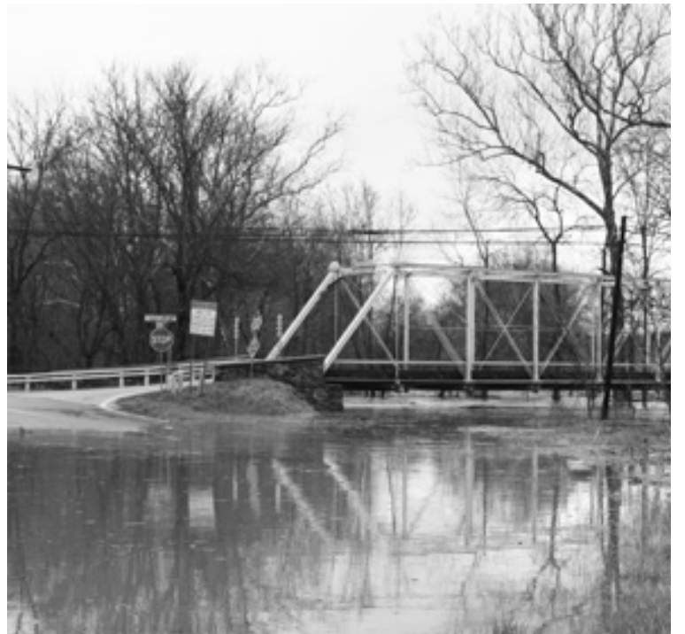
Tom's Creek flooding at Tom's Creek Bridge
