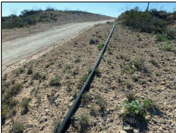
Figure 5. Road and pipeline impacting CC002.
