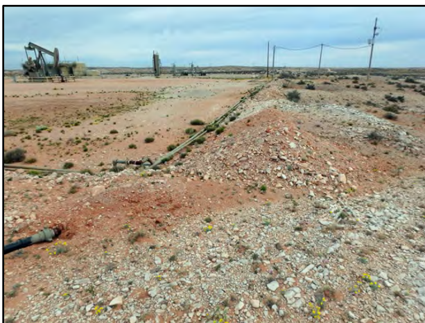
Figure 9. State land well pad at RL037.
