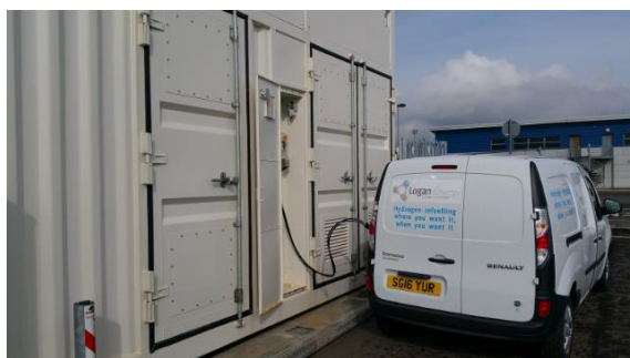
Figure 3.2.1: One of the Renault Kangoo hydrogen-electric vans deployed in Levenmouth (Image copyright Logan Energy)
