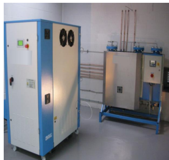
Figure 4.2.1.1(b) Alkaline Electrolyser
