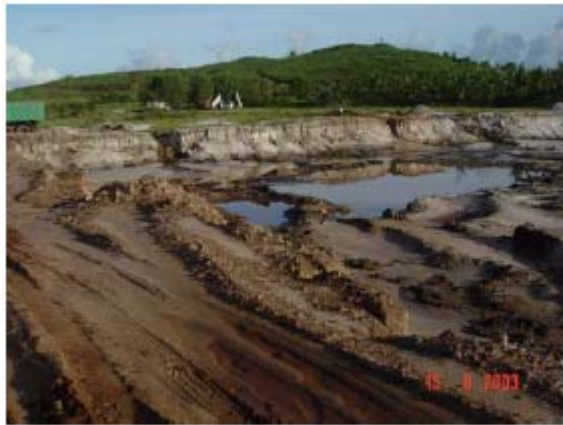
Figure 3. Land Removal in Sihanoukville, and a lot of sediments were washed away the most to the nearby reefs.
