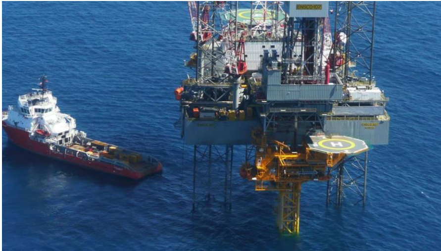
Figure 3 Example of jack-up MODU cantilevered over the Kupe WHP
