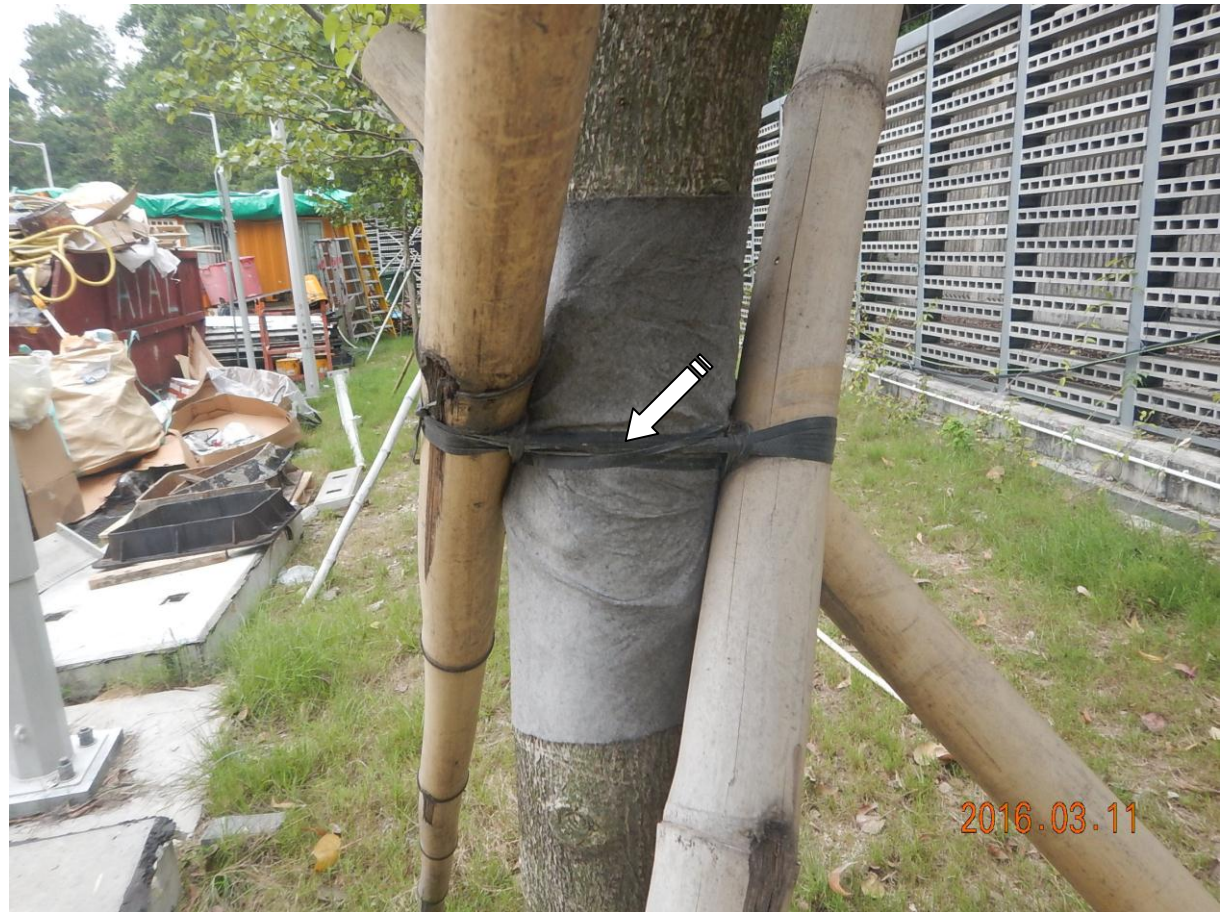
Photo no. G-08: The non-abrasive nylon rope for securing the trees was observed to be too tight.
