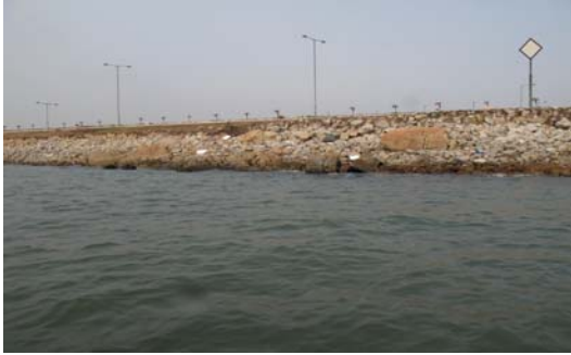
Artificial Slopping Boulders at D1
