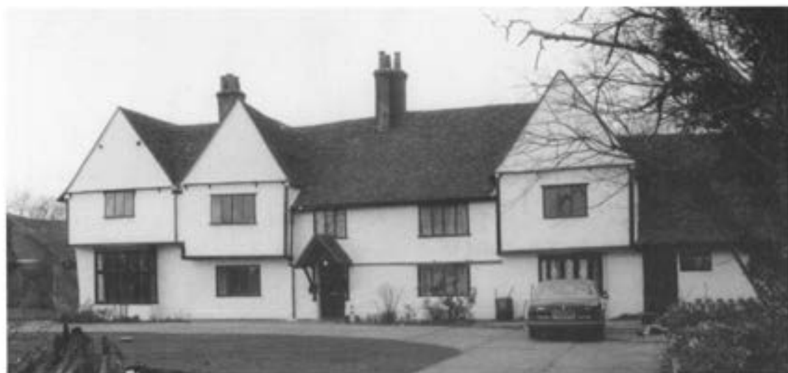
Plate 2 Nether Hall farmhouse.
