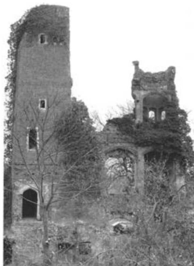
Plate 5 The north side of the stair tower (Nicolette Hallett).
