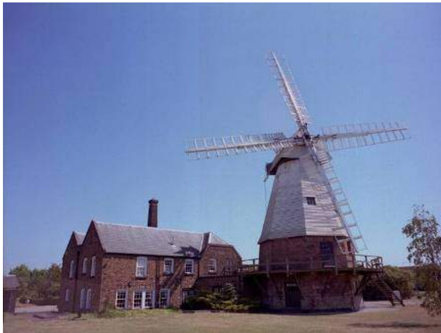
Photograph of Baker Street Smock and Steam Mills
