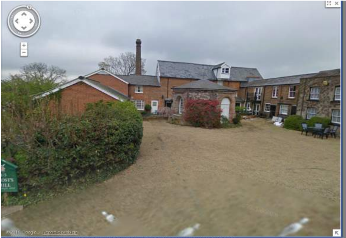
Photograph of Frost's Mill Halstead (Google Maps Street view, retrieved on August 2011)
