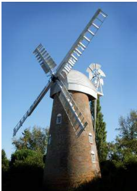
Figure 6 Photograph of Stock Tower Mill
