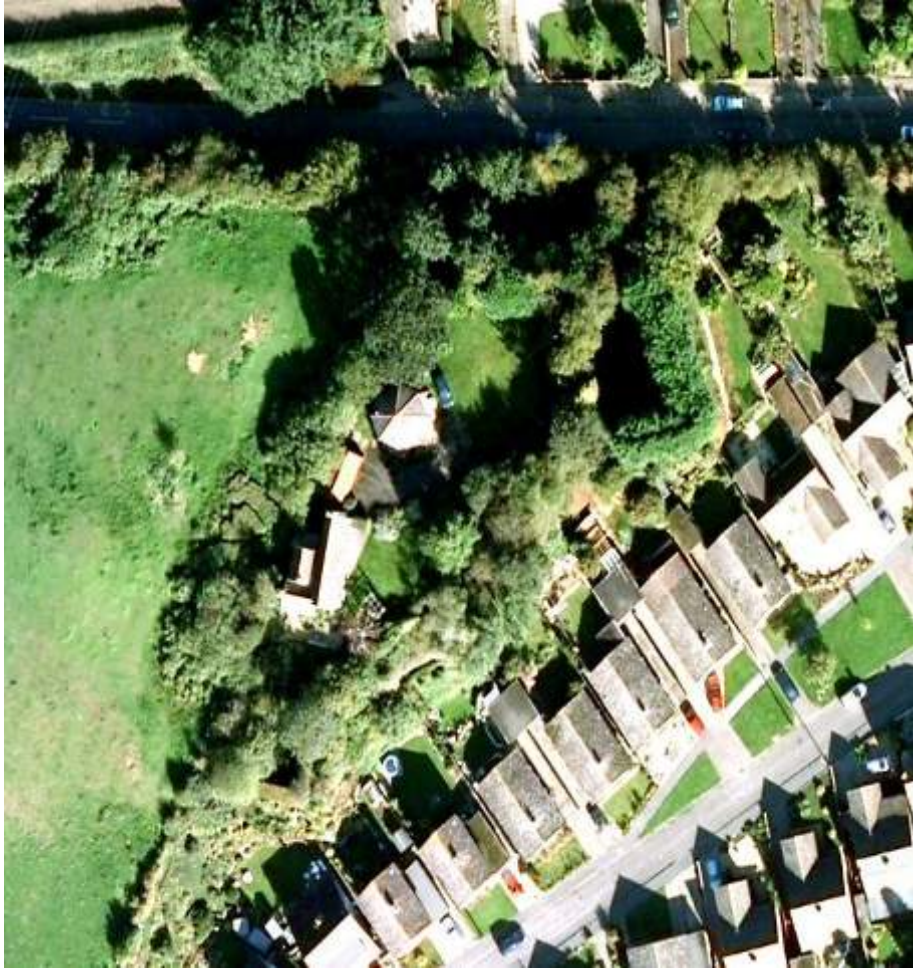
Photograph of Bulmer Smock Mill Base (Google Maps Street view, retrieved on August 2011)
