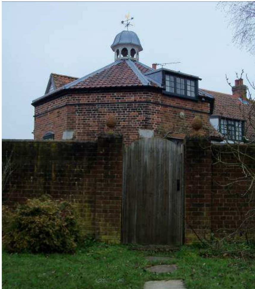
Photograph of Wimbish Tye Green Smock Mill Base
