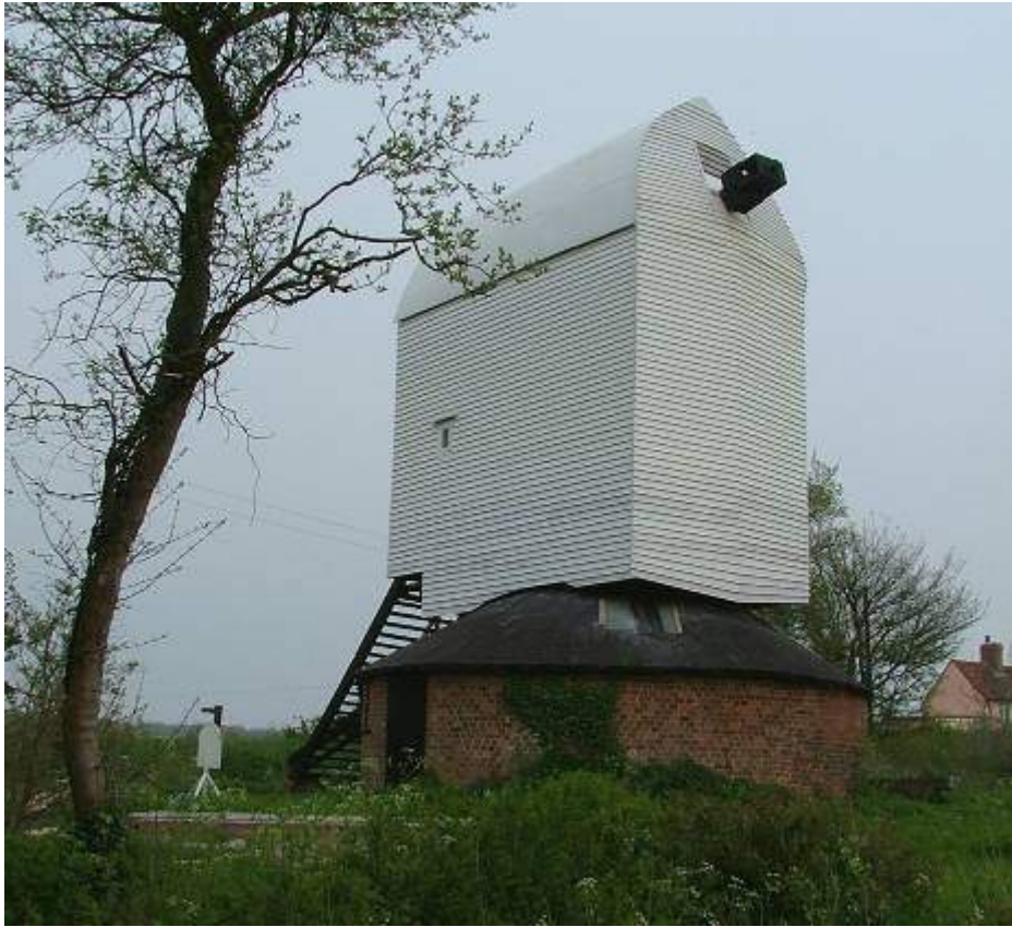
Photograph of Ashdon Post Mill (Google Maps Street view, retrieved on August 2011)
