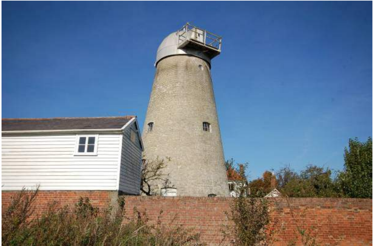
Photograph of White Roding Tower Mill(Google Maps Street view, retrieved on August 2011)
