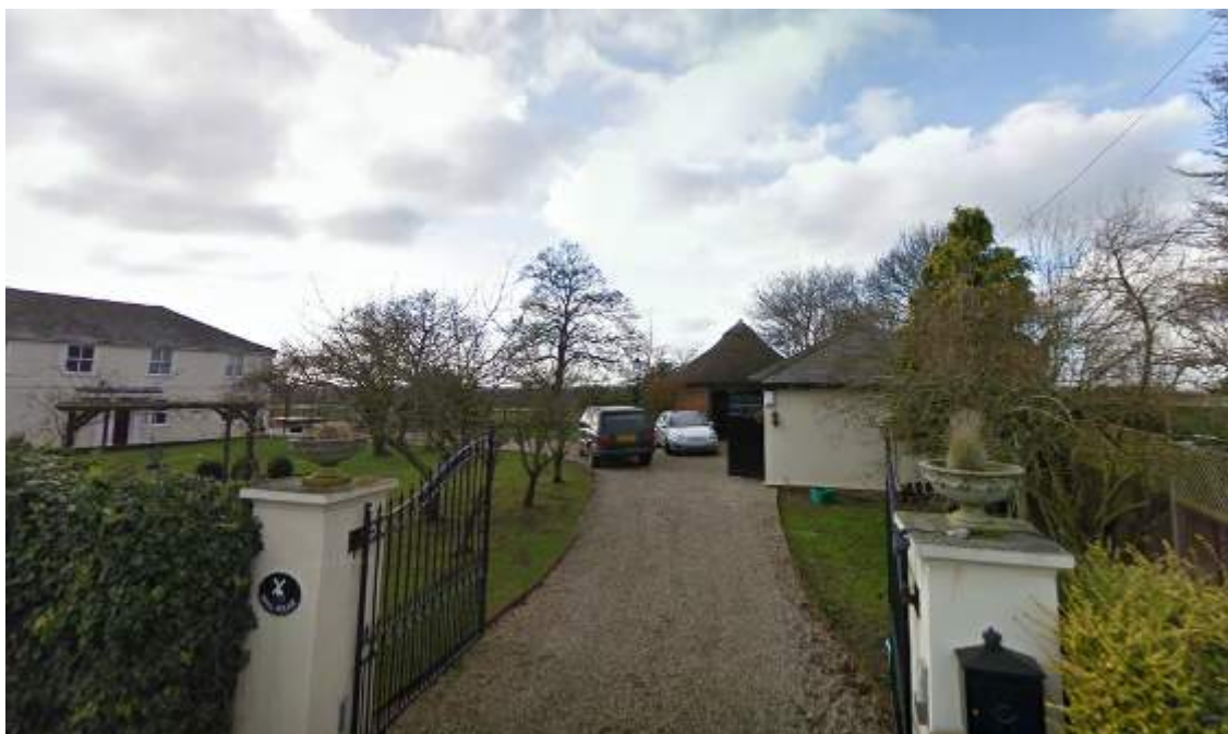
Photograph of Mashbury Smock Mill Base Windmill Roundhouse (Google Maps Street view, retrieved on August 2011)
