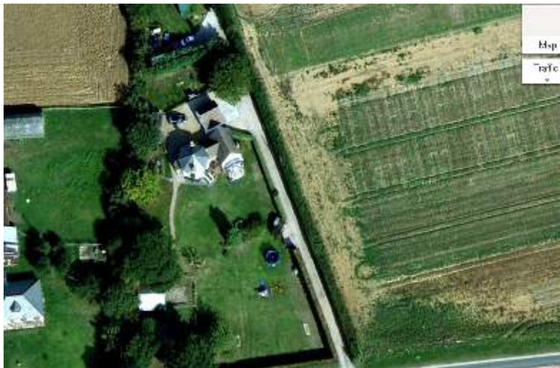
Photograph of Throws Mill Roundhouse (Google Maps Street view, retrieved on August 2011)
