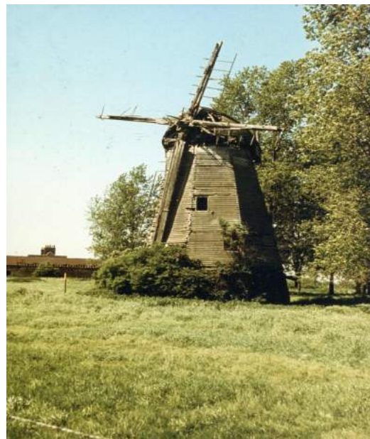
Figure 8 South Ockendon Smock Mill
