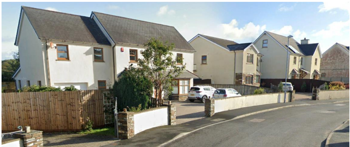
Photo 8 – use of render and stone detailing to Maes-y-Wennol properties
