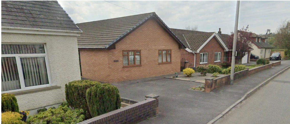
Photo 9 – use of face brick upon bungalows fronting the B road west of the Square and public houses
