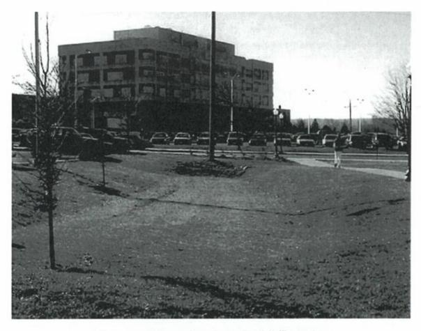
Figure 10.1. Typical Dry Swale in commercial/office setting
