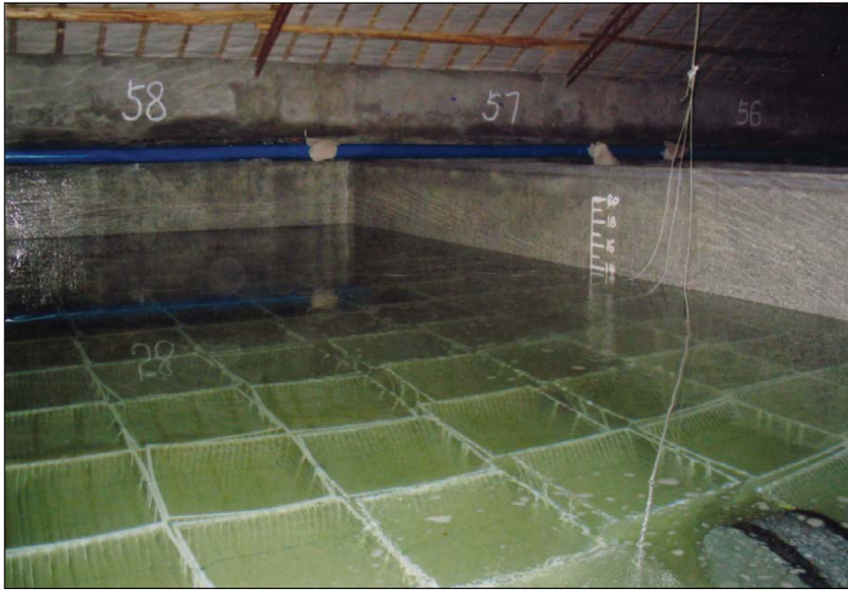
Figure 4. Installation of settlement plates.
