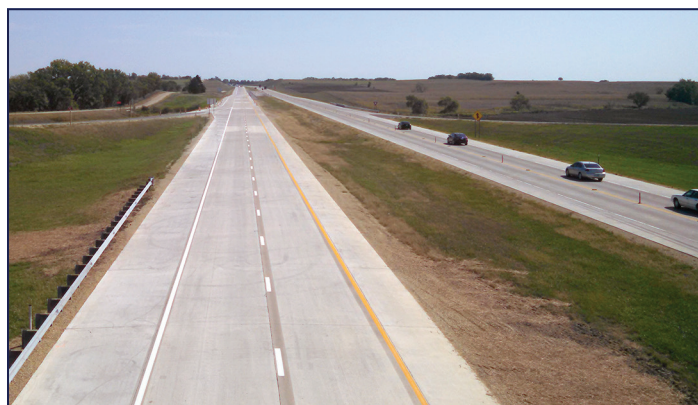
I-70 open to traffic (ACPA)
