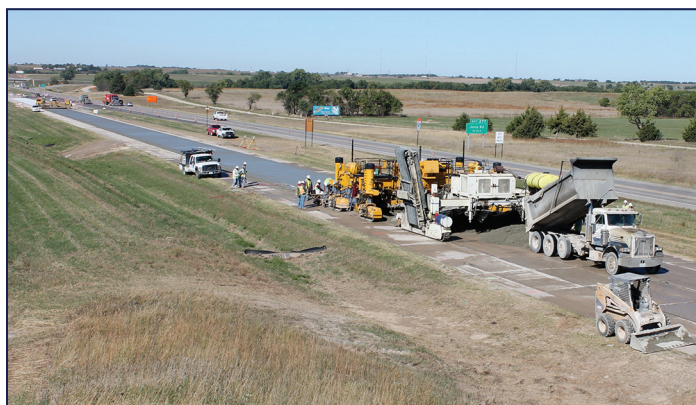
Placing 3½-inch concrete overlay (ACPA)
