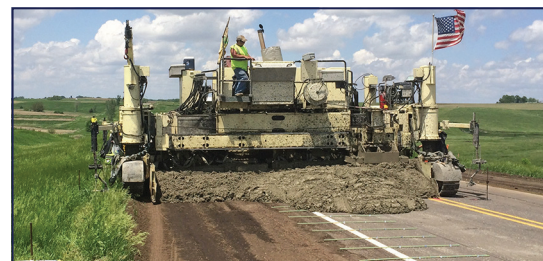
Placing 6-inch concrete overlay on geotextile (Iowa DOT)
