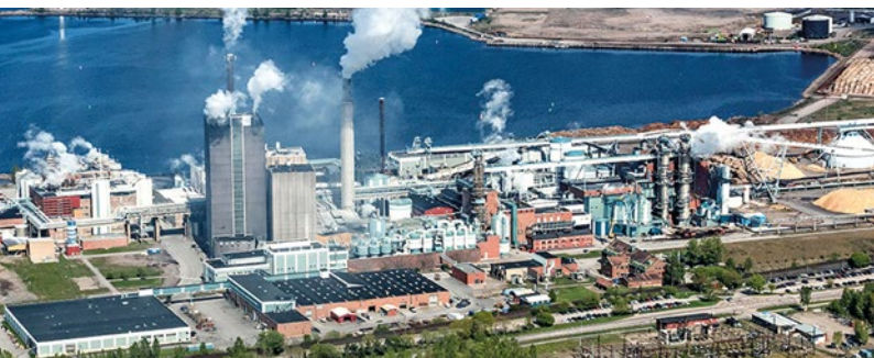
StoraEnso Skutskär Mill in eastern Sweden is a modern pulp mill that primarily produces fluff pulp
