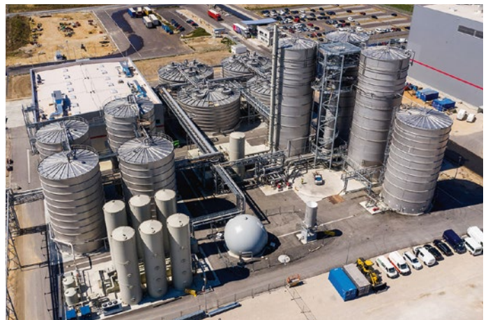
The new type of circulating water treatment plant of PM3 treats the process water used and returns it to the closed water cycle of the paper production.
