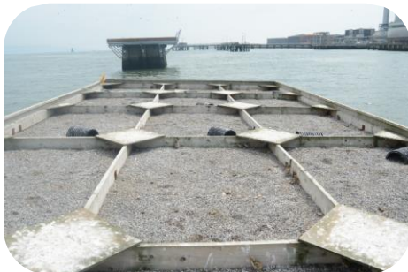
Figure i: Wooden edging and wooden 'roofs' and plastic tubes for shelter for Terns and their chicks at Dublin Port specially constructed platform.
