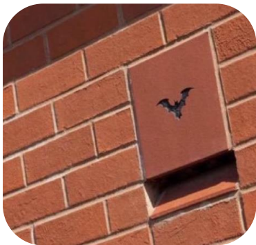
Figure 13: An integrated bat box in a building
