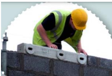
Figure 3: An integrated Swift nesting box in a building
