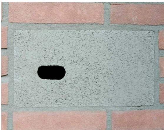
Figure 2: Swift nest box placed on outside of building under eaves
