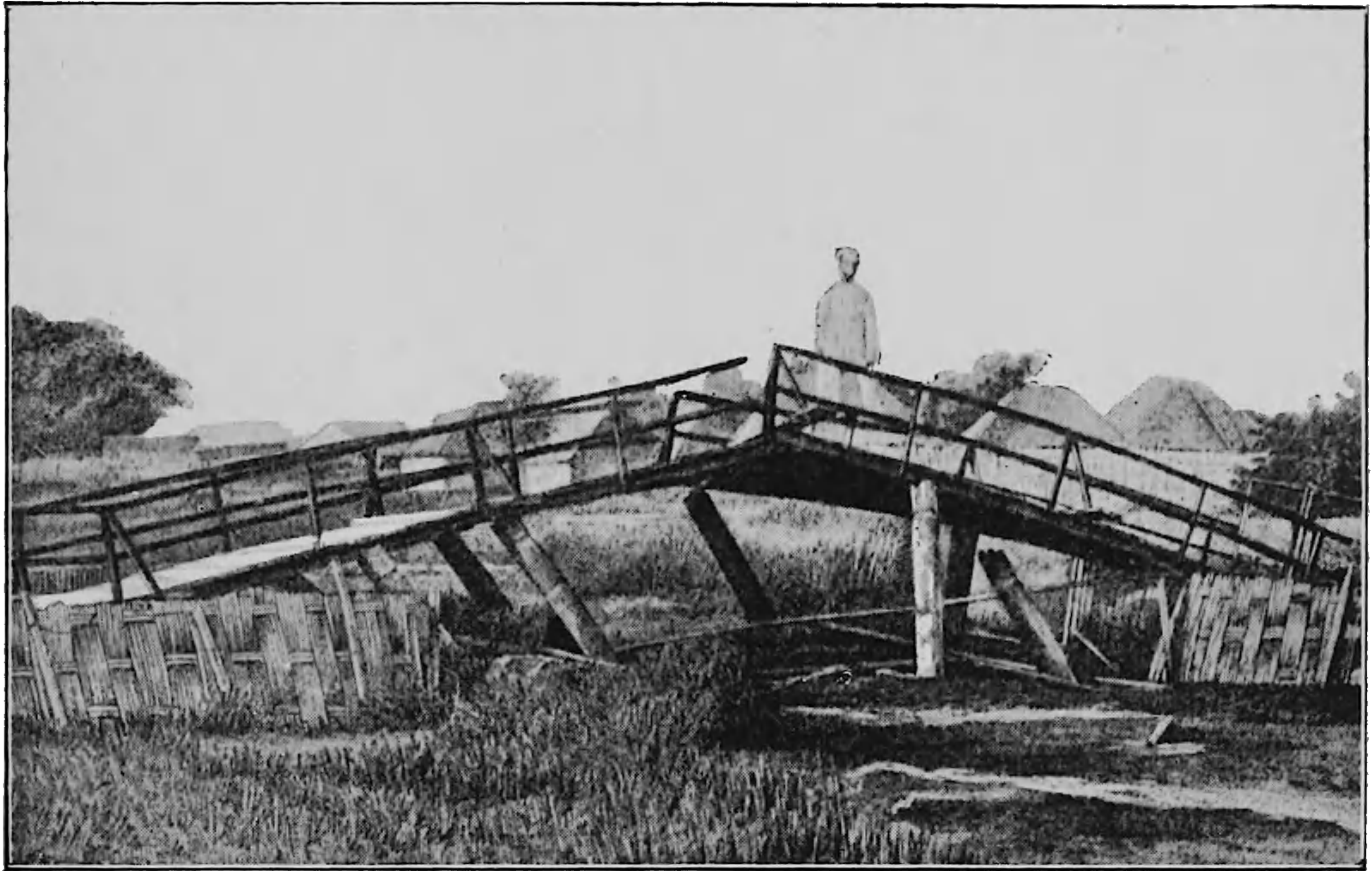
BRIDGE ACROSS NALLAH AT HALDIBARI
