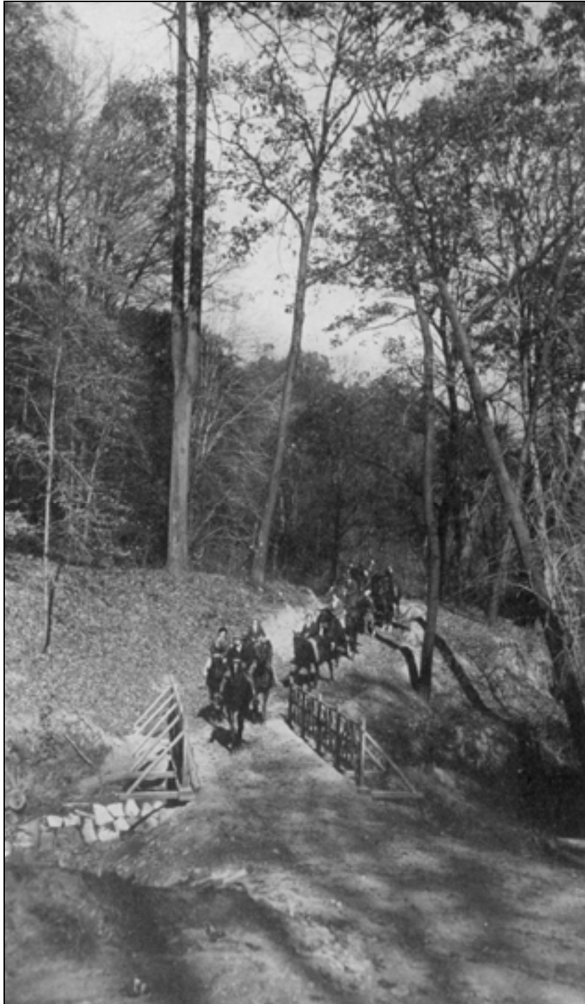
Figure II.14 View of the second footbridge constructed across the St. Mary's River. This footbridge was constructed to accommodate horseback riders from the nearby Riding Academy and provide access to the bridle path in Foster Park. Courtesy Fort Wayne Parks and Recreation. (R- FWP-FOS-PD-Brd-Rpt-BridlePath-1933-pg13.jpg)
