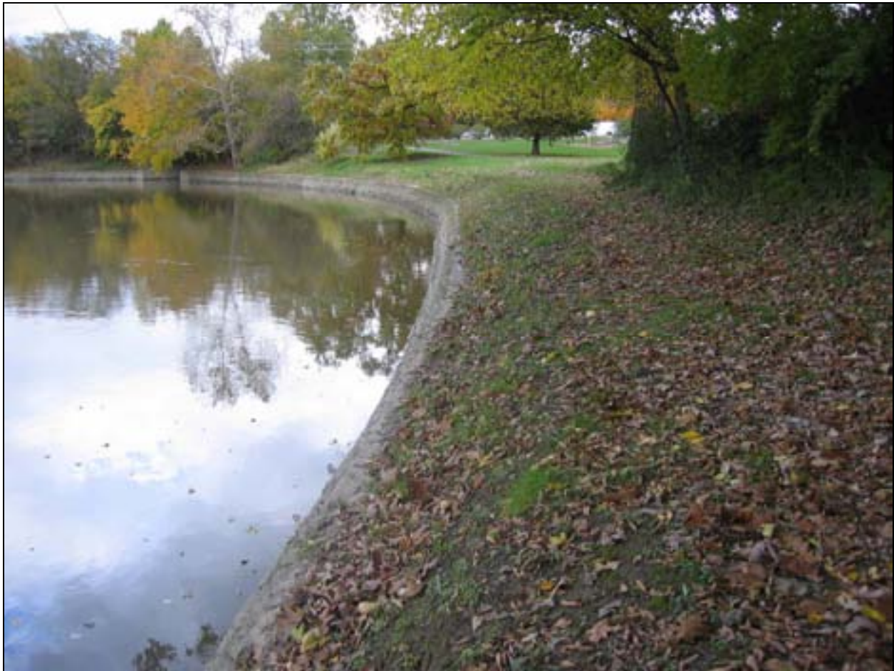
Figure IV.10 View looking east along the St. Mary's River. A simple stone and mortar retaining wall lines the eastern river edge, stabilizing the bank and preventing erosion. An asphalt pedestrian path is visible in the background, framed by two park trees. Courtesy Heritage Landscapes. (R- FWP-FOS-VT-0014.jpg)
