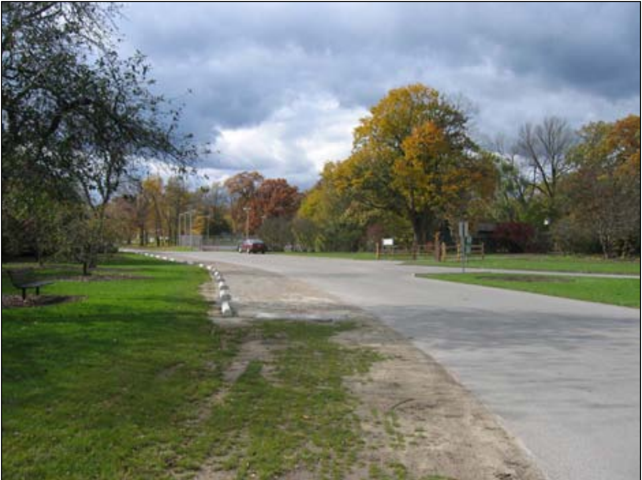
Figure IV.5 View looking west into Landscape Area 2. The gently curving park entrance drive with bordering gravel parking areas defines a portion of the southern edge of the area. Park features in this area include sports courts, a playground, and the garden which are set within open turf under tree canopies. Courtesy Heritage Landscapes. (R- FWP-FOS-VT-0024.jpg)
