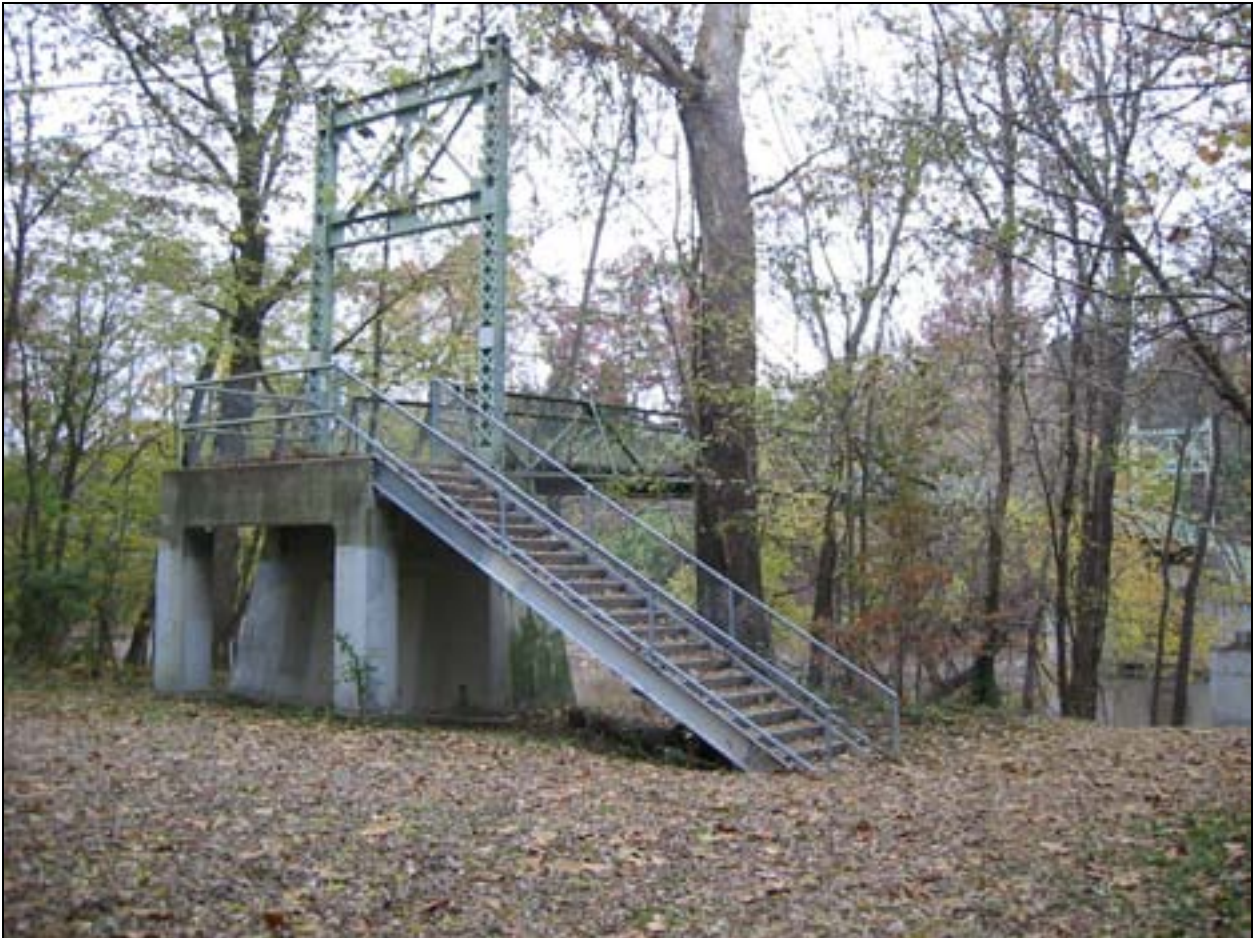
Figure IV.21 View looking toward the steel and concrete park footbridge. The bridge crosses the St. Mary's River in the northern section of Landscape Area 4. Originally constructed to provide safe crossing between Indian Village and Foster Park, the footbridge continues to be widely used for safe and easy park access. The bridge connects to the meandering woodland path in Landscape Area 4. Courtesy Heritage Landscapes. (R- FWP-FOS-CT- (166).jpg)
