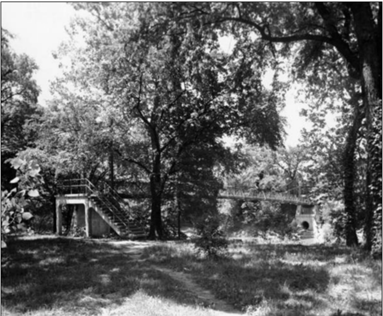
Figure II.13 View of the concrete and steel footbridge constructed across the St. Mary's River to connect Foster Park with the Indian Village, located north of Foster Park on the opposite river bank. Note also the narrow compacted earth path leading to the bridge and the surrounding vegetation along the river bank. Courtesy Allen County Public Library, Genealogy Division. (R- FWP-ALCA-Foster-Footer-Bridge-ND.jpg)
