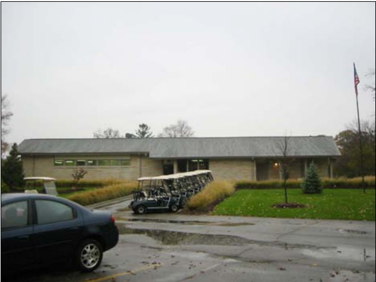
Figure IV.14 View looking at the east façade of the golf clubhouse. The clubhouse is situated at the northwest edge of the golf course parking lot. An asphalt path links the parking area with the covered entry. Other landscape features shows include mulched planting beds, ornamental plantings, and a flagpole. Courtesy Heritage Landscapes. (R- FWP-FOS-CT- (345).jpg)
