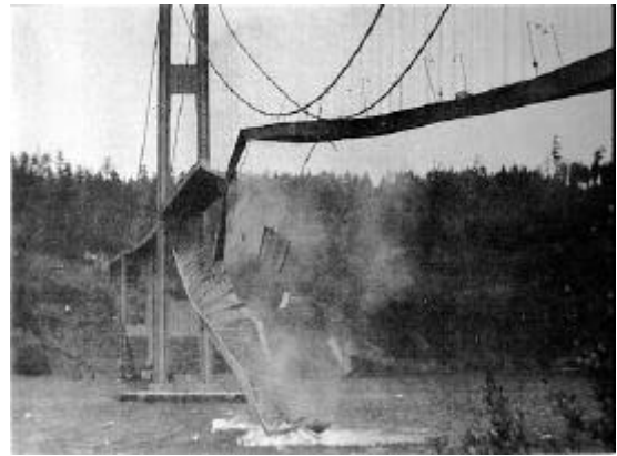
Collapse of Tacoma Narrows Bridge due to Lock On Effects 10
