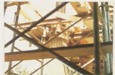
Capital to column on south elevation
