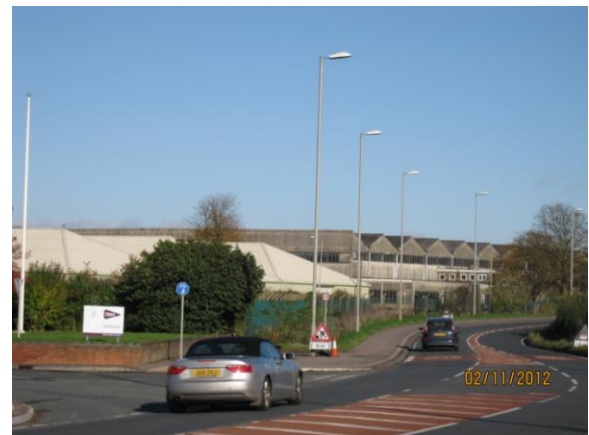
View from A38 of MOD site at Ashchurch.
