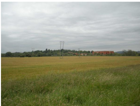
View across flood meadows towards Water Treatment Works.
