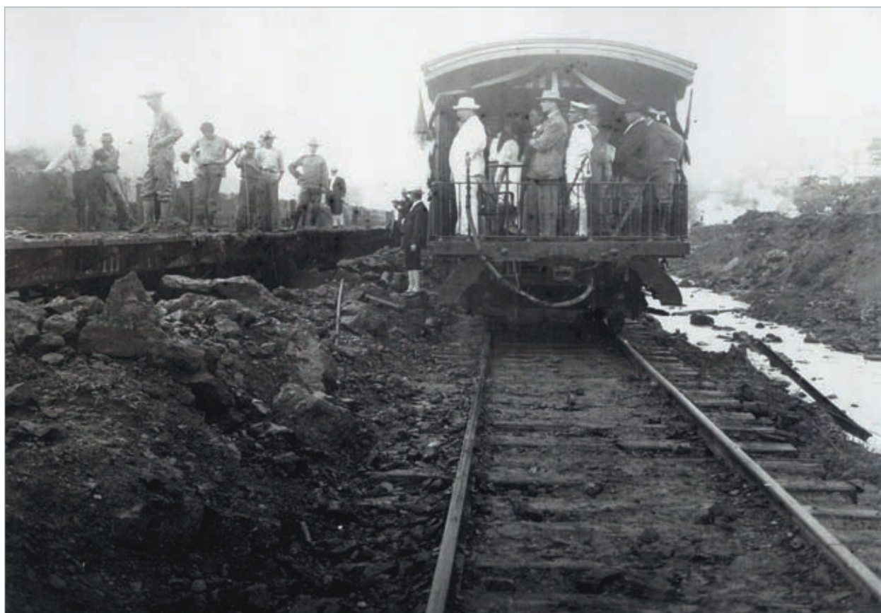
PRESIDENT THEODORE ROOSEVELT INSPECTING CANAL WORK FROM RAILROAD COACH
