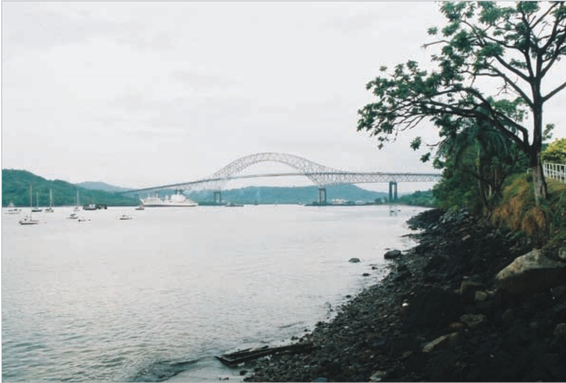
Thatcher Bridge. (Photo by Peter L. Weaver)
