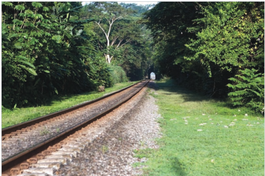
Tunnel at Miraflores. (Photo by Gerald P. Bauer)
