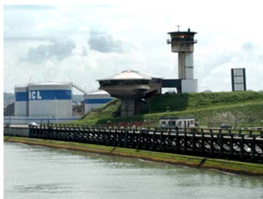
Boulogne Port Control Tower
