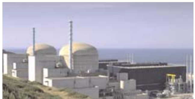
Flamanville Nuclear Power Station
