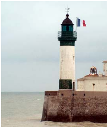
Le Treport Light (West Breakwater)
