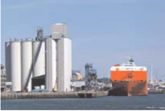
Eastern Docks Silo
