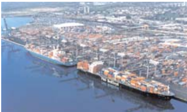
Southampton Container Terminal
