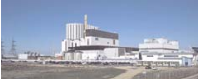
Dungeness Nuclear Power Station
