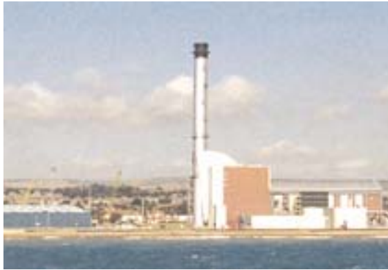
Shoreham Power Station
