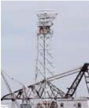
Admiralty Jetty Radar Tower
