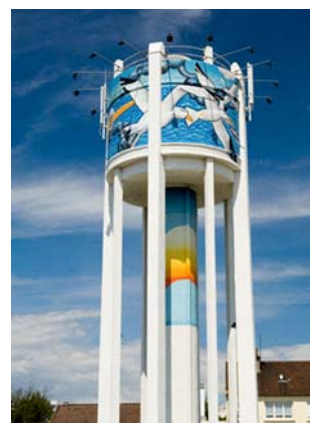
Calais—Bleriot-Plage water tower
