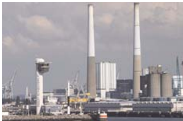
Le Havre (Port Control tower and power station)
