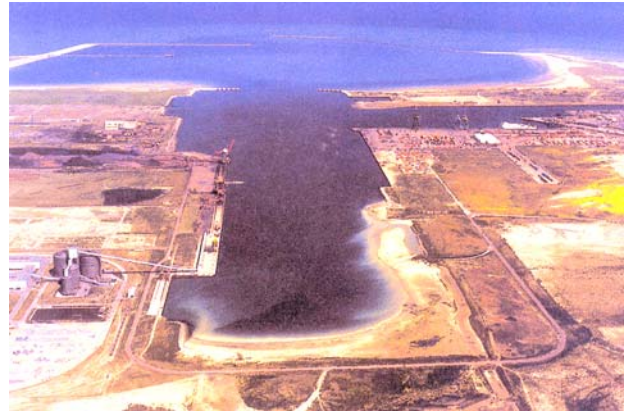
Dunkerque—Port Ouest from S
