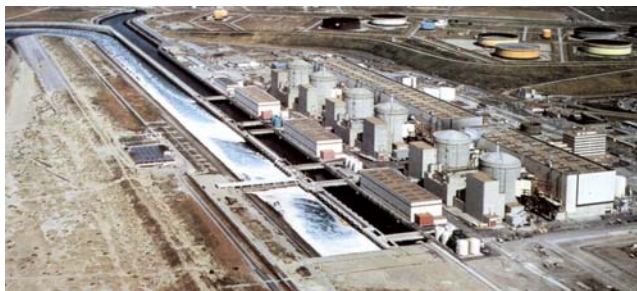
Gravelines Nuclear Power Station
