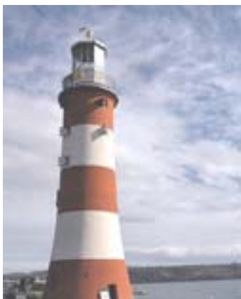
Smeaton Tower (disused)
