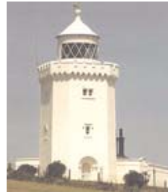
South Foreland Light Tower (disused)
