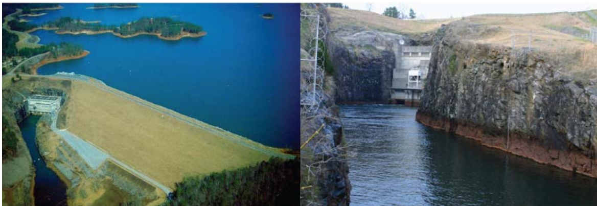
Plate 3. Left – Lake Lanier and Buford Falls Dam, U.S. Army Corps of Engineers Digital Visual Library ( http://eportal.usace.army.mil/sites/DVL/default.aspx ). Right – Close-up of the dam ( http://georgiainfo.galileo.usg.edu/hoochbuford1.htm ); photo by J. Kundell, used with permission.
