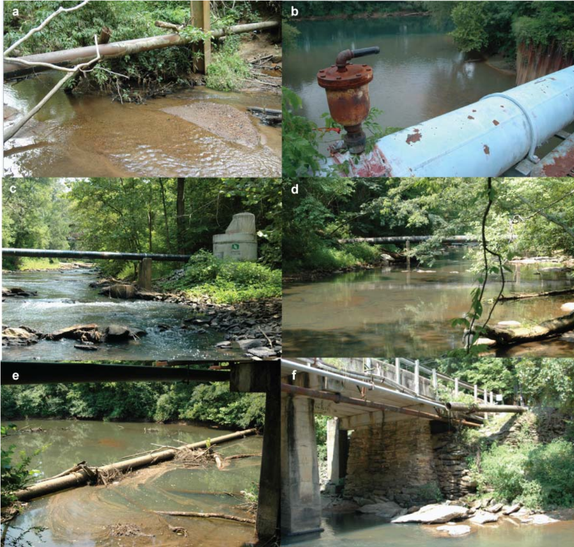
Plate 20. Examples of the numerous sewer pipes that traverse or empty into park waters, including (a) Gold Branch – Willeo Creek, (b) Suwanee Creek – turbid Suwanee Creek at its confluence with the Chattahoochee River, (c-e) Vickery Creek, and (f) Cochran Shoals showing straight-pipe runoff into the Chattahoochee River. Photos by E. Morris, 2008.
