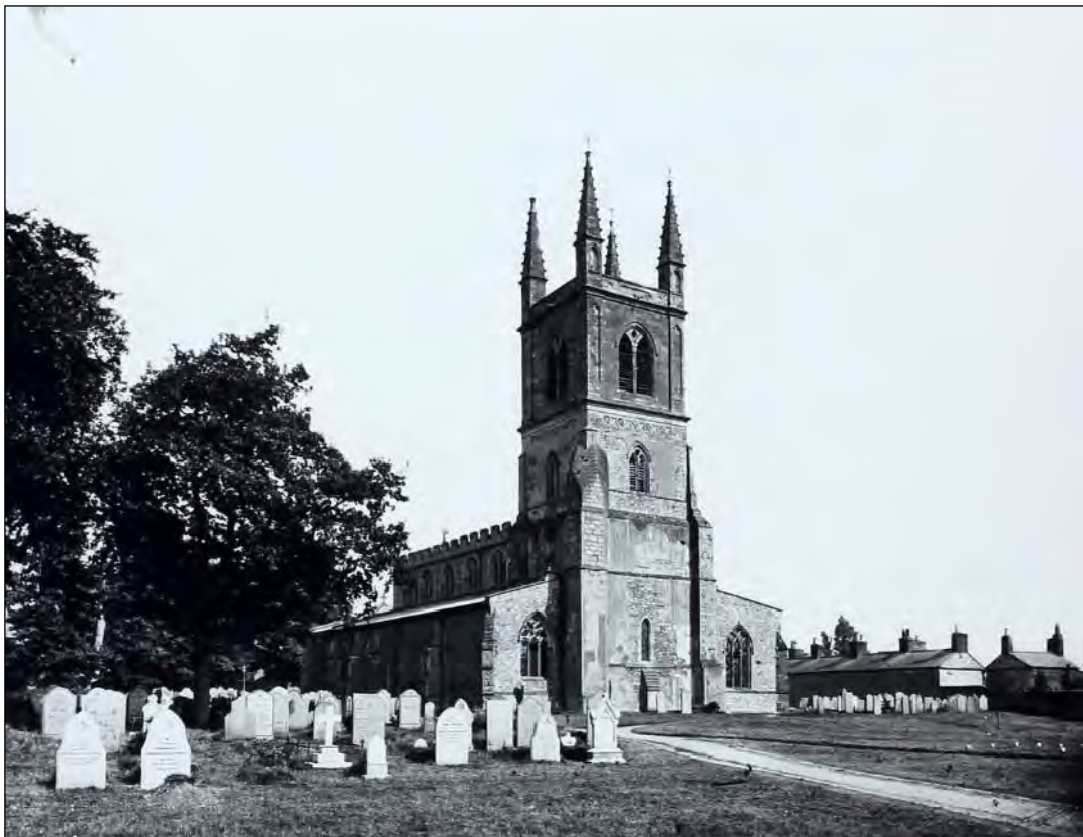
Photo 13 1885 view of St Mary's from the NW corner of its churchyard
