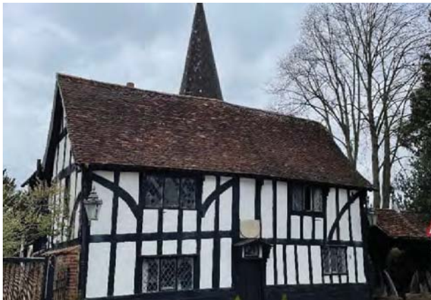
3 Traditional timber framed building, Churchgate Street
