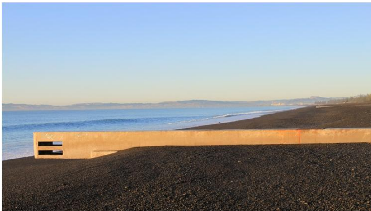
Figure 7.5. Storm water outfall adjacent Marine Parade – Napier City.
