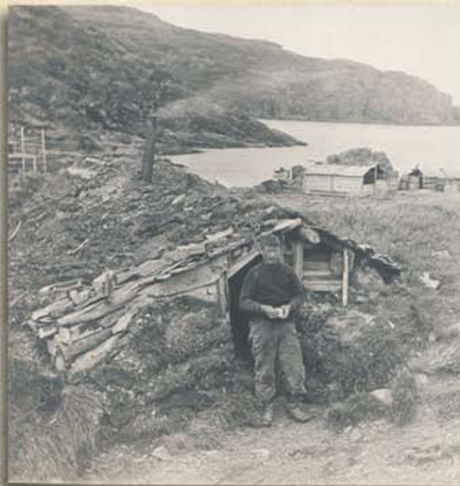
3.45 Using what's available Sod-covered dwellings were common in Labrador due to a lack of timber in some areas.
