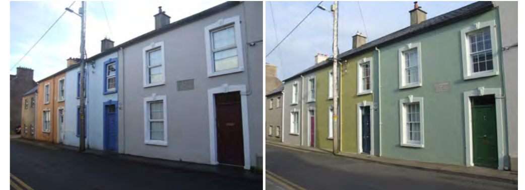
Terraced houses along The Mall (including the birthplace of poet William Allingham) that benefitted under the award-winning Ballyshannon Historic Towns Initiative. Photo: Joseph Gallagher
