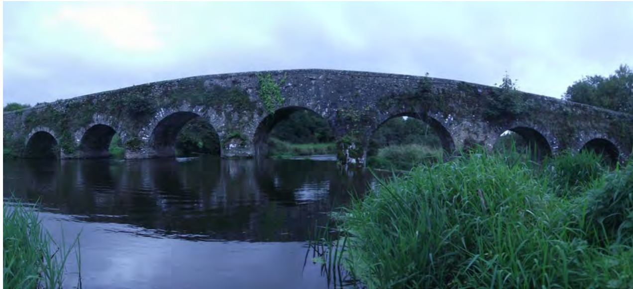
The medieval bridge in Glanworth. Photo: Cork County Council Heritage Unit
