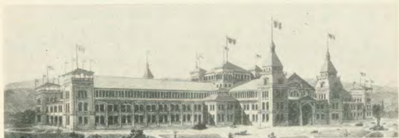
MINING AND INDUSTRIAL EXPOSITION BUILDING, 1882
