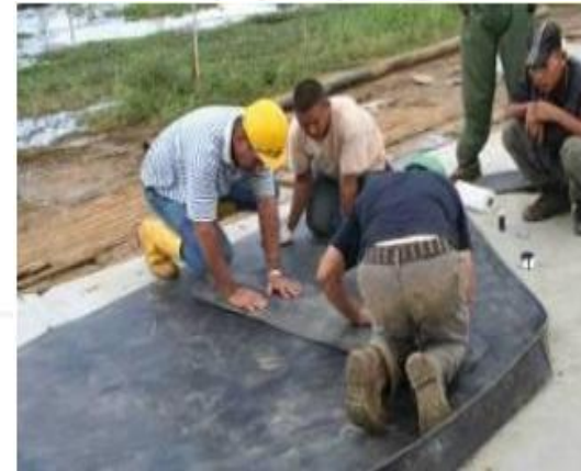
Skirts being repaired on site
