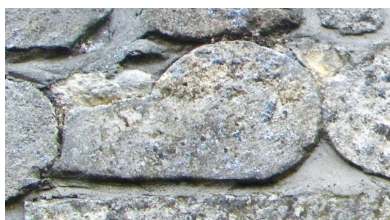
One of the 'whistle' stones that has been reused in the east end of Hyde House. William Bethell built the house adjacent to the demolished Abbey buildings in the second part of the 16th century. The shaft is oval rather than circular and the tongue is at 135 degrees from the shaft.
