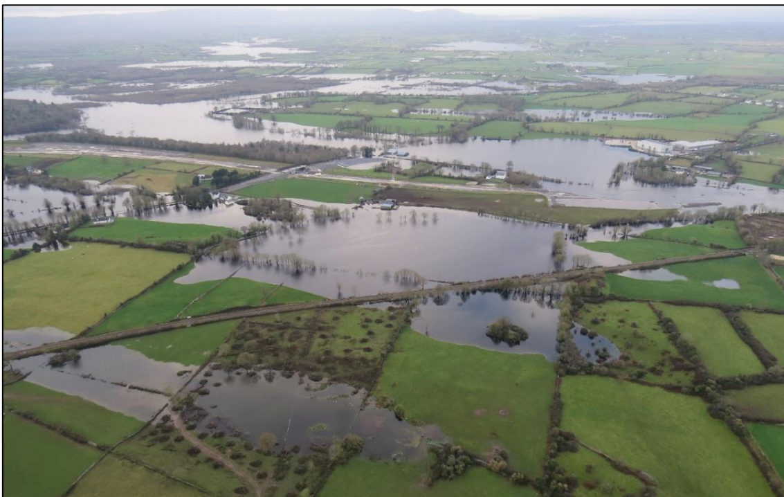
Figure 37: Groundwater flooding in the vicinity of the Coole Complex during January 2016 (Image courtesy OPW).
