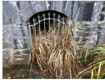
The Double well closest to the pump house: iron staining is visible on the ground near the well, so this may be the chalybeate well.
