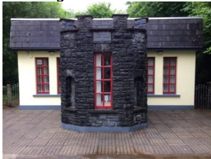
The old pump house near the Double wells, which is now a library (note the two external taps in the alcoves on the tower like entrance to the building).
