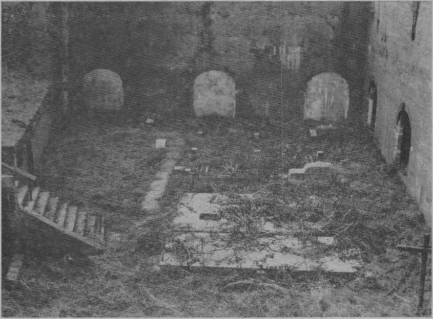
Figure 13.—Mining control room, Fort Washington, Md.
