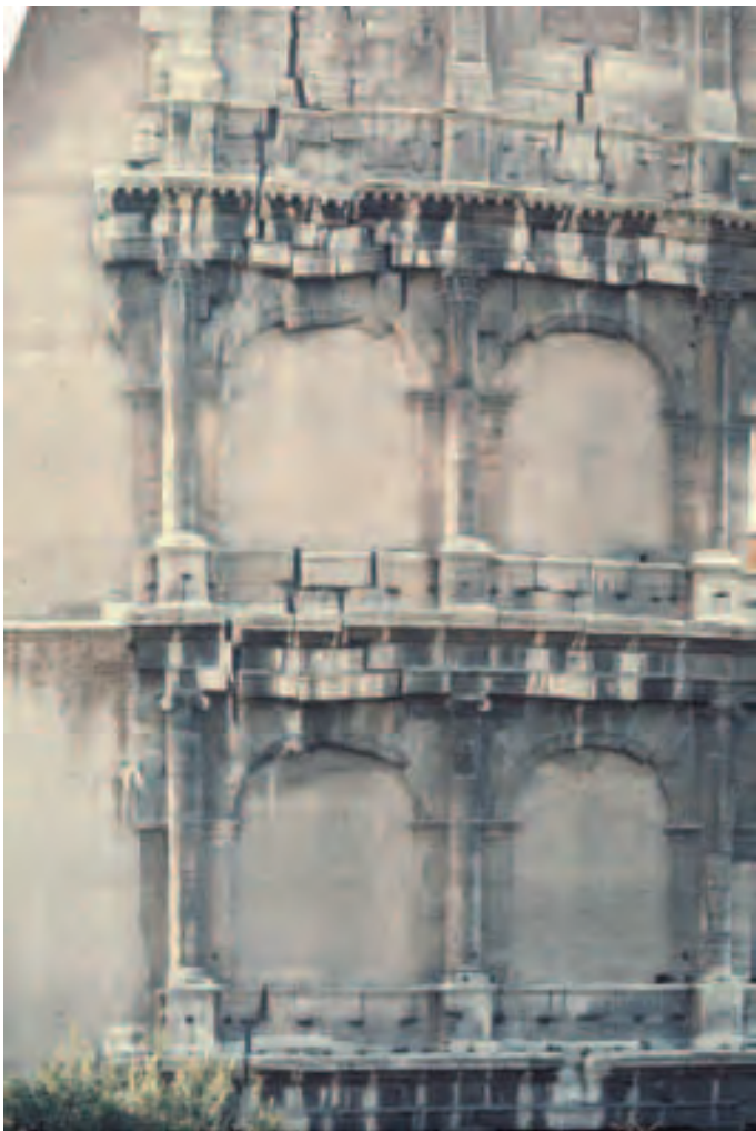
Figure 92. The Colosseum. The brick buttress built to support the east wall; a detail
