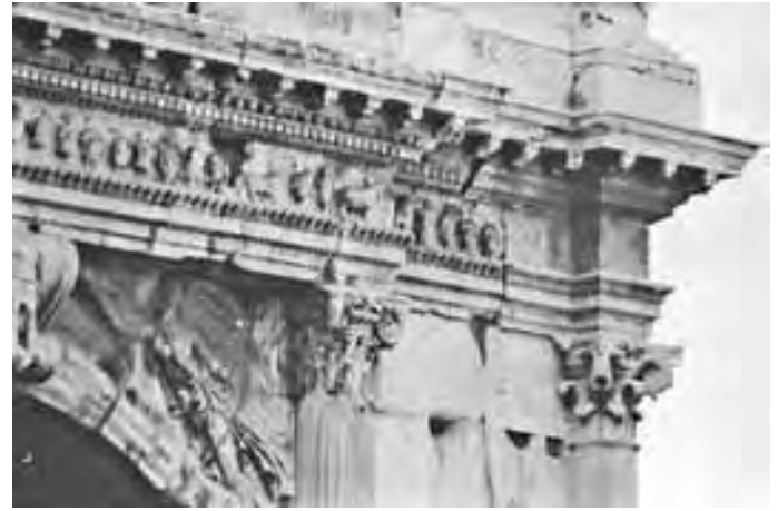
Figure 108. Arch of Titus, detail showing the distinction between original (in marble) and new (in travertine and simplified details)
