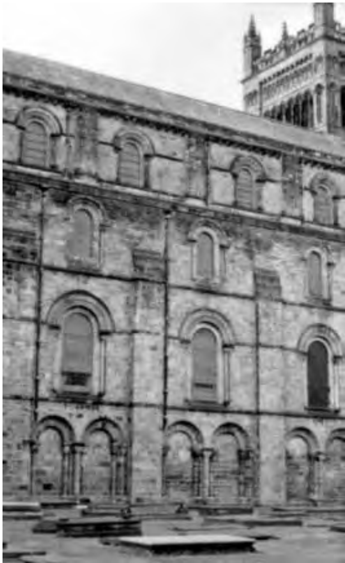
Figure 165. Durham Cathedral, north elevation after restoration
