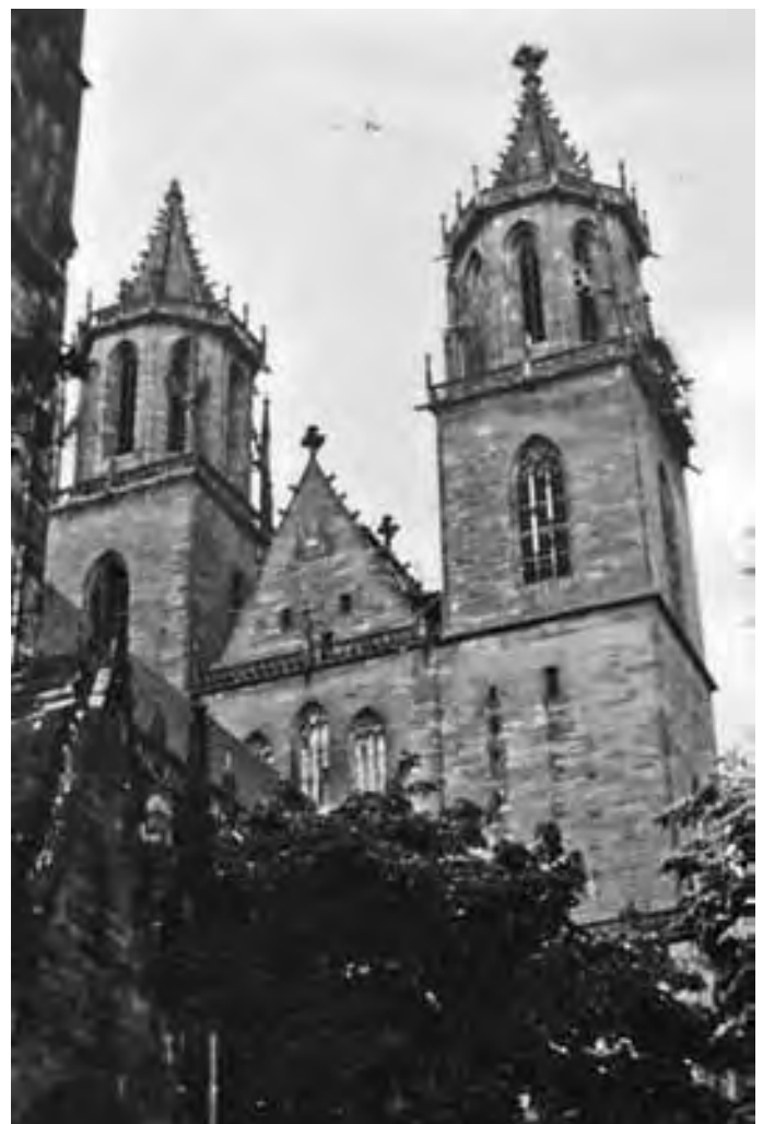
Figure 186. Magdeburg Cathedral, western towers in 1979
