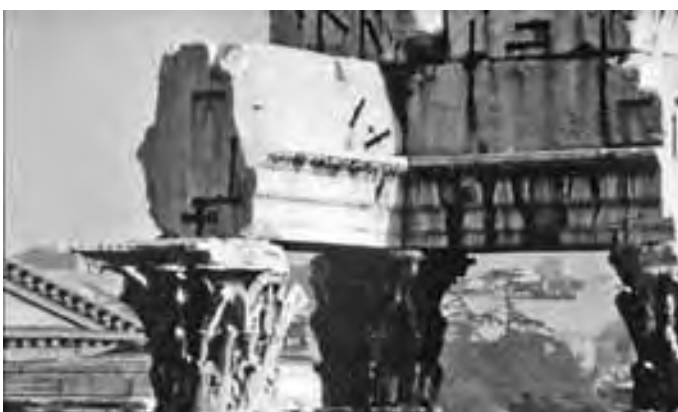
Figure 97. The Temple of Vespasian and Titus: a detail of the architrave after the 19th-century restoration using metal cramps
