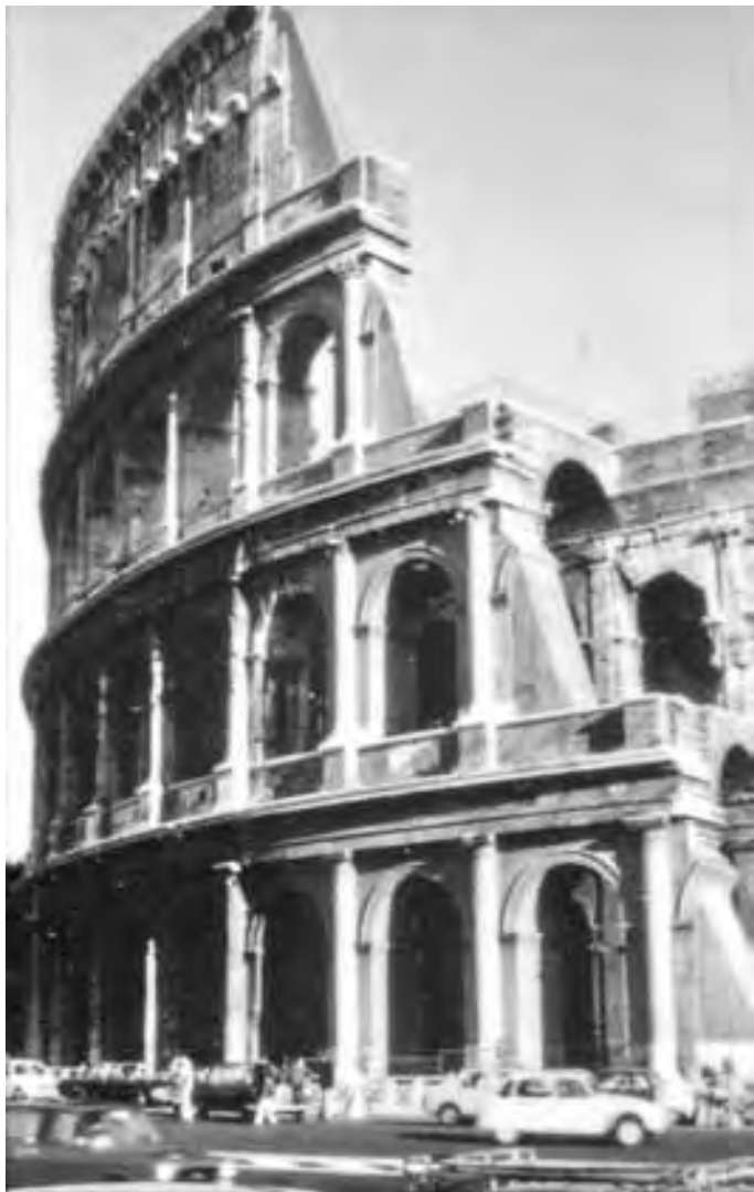
Figure 113. The Colosseum after the construction of the buttress by Valadier for the consolidation of the west wall
