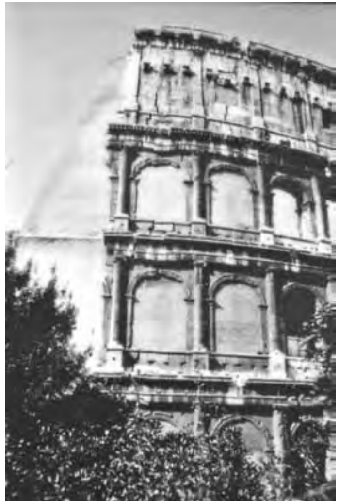
Figure 91. The Colosseum. The brick buttress built by R. Stern in 1806-07 to consolidate the east wall
