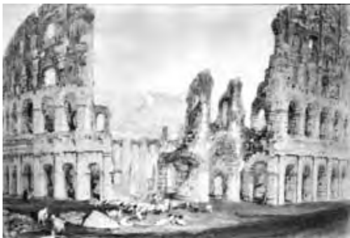
Figure 114. The Colosseum: south wall before restoration (Turner)
