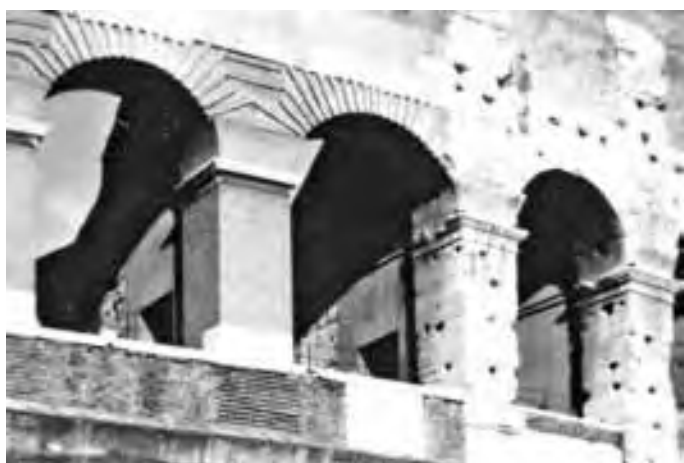
Figure 115. The Colosseum: south wall; detail of the part restored by L. Canina
