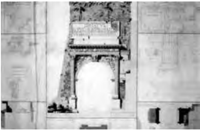
Figure 102. Guënepin (1810): the Arch of Titus, Rome, showing the condition of the monument before beginning of the restoration
