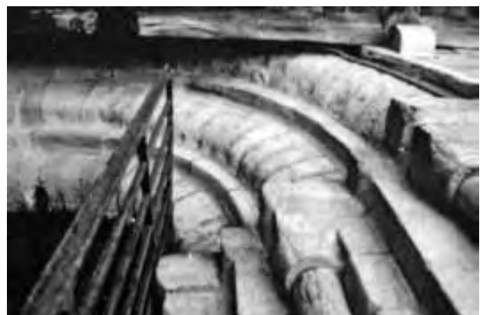
Figure 142. Durham Cathedral, entrance from the cloister; detail showing the effect of scraping the surface
