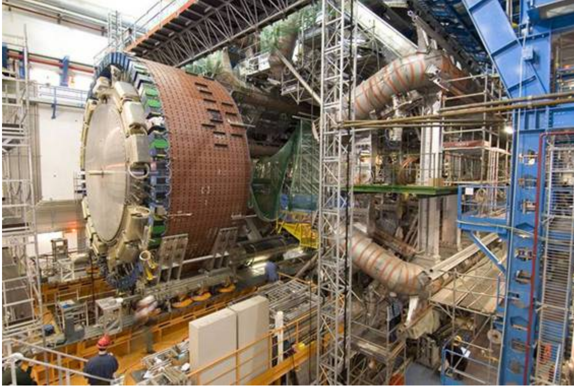
A view of the ATLAS cavern in March 2006: The Tilecal Barrel built at IFAE (brown cylinder on the left) is being inserted into the huge toroidal magnet vacuum vessels, built by a company in Spain. Two of the vessels are visible on the right hand side of the figure (structures with brown stripes). The superconducting coils of the barrel toroidal magnet system are inside these vessels.
