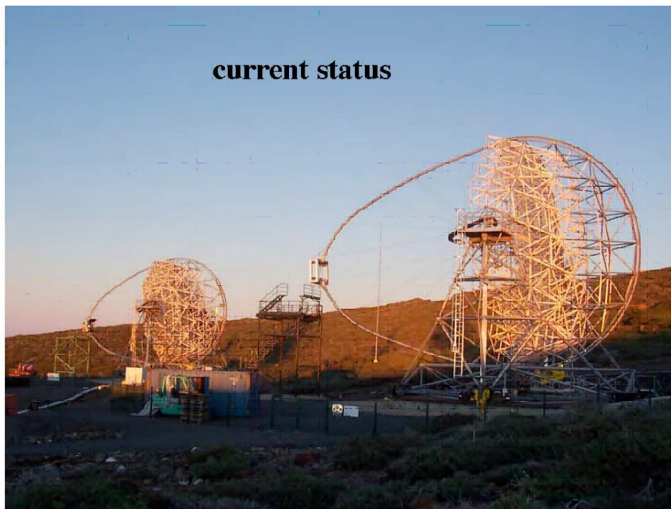
The two MAGIC telescopes in Nov. 2006. The nearer instrument is MAGIC-II, undergoing installation of its main components at the time of the picture.
