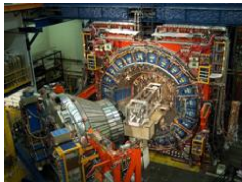
CDF during the installation of the Silicon Detector into the tracking chamber.
