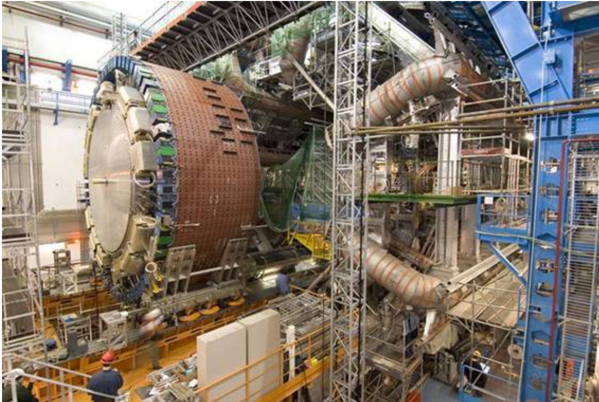
A view of the ATLAS cavern in March 2006. The Tilecal Barrel built at IFAE (brown cylinder on the left) is being inserted into the huge toroidal magnet vacuum vessels, built in Spain. Two of the eight vessels (with brown stripes) are visible on the right hand side of the figure; they enclose the superconducting coils of the barrel toroidal magnet system.
