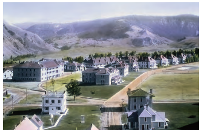
The aging irrigation system used to water the historic lawns of Fort Yellowstone and Mammoth Hot Springs, pictured here in 1916, was upgraded in 2012.
