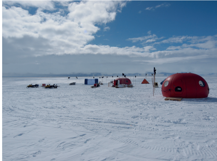
Fig. 3.2.8.3: Facilities of the Drescher ice camp. In order to guard against strong snowdrifts, igloos, tents, and generators were lined-up across the main easterly wind direction. Photo: Horst Bornemann, AWI
