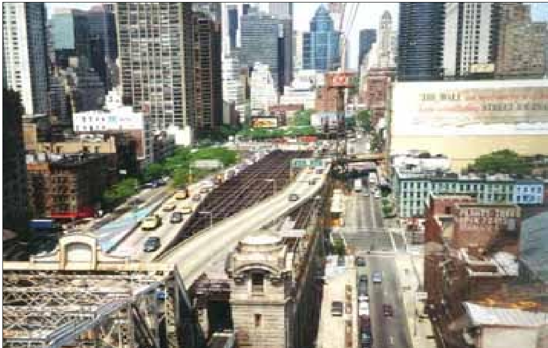
The Queensboro Bridge ramp between 59 th and 60 th Street ending at Second Avenue. Looking west.
