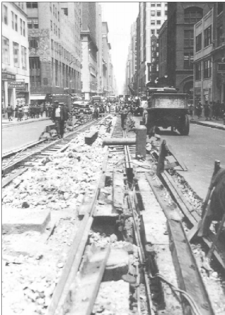
Picture 2.1-2: Tearing up Trolley Tracks
