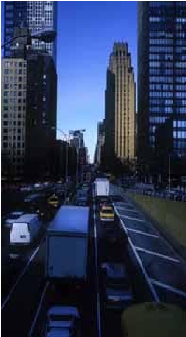
First Avenue at 48 th Street. Looking north. Exit of the UN underpass, originally designed for two-way traffic.
