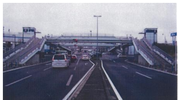
(b) Road at improved are after earthquake.
