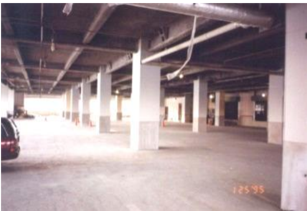
(b) Parking area in the building.
