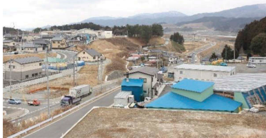
Figure 49. New town center at top of hill (Rikuzen-Takata, March 2017).
