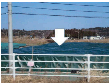
Figure 75. Piles of plastic bags to store radioactively contaminated surface soil around the power plant (January 15th, 2019).
