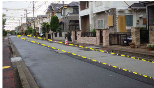
Figure 61. Construction of underground wall under street by mechanical mixing.
