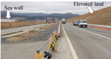
Figure 50. Raising ground level by 15 m in former town area (Rikuzen-Takata).
