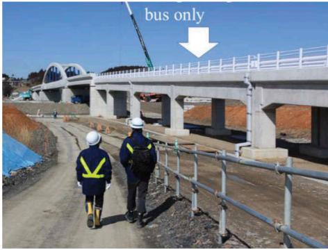
Figure 51. Reconstruction of local public transport by bus rapid transit (Kesen-numa).
