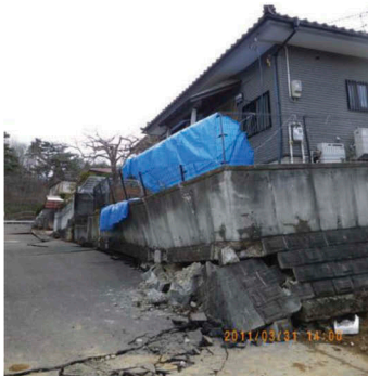
Figure 19. Seismic damage of residential land in the suburban hill area of Sendai.
