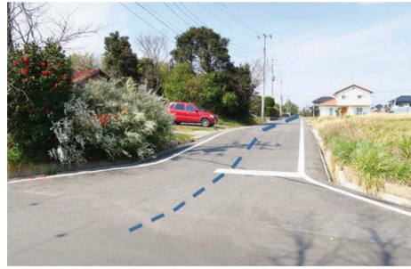
Figure 54. Hinode District of Itako City where ground water is drained by gravity flow through installed pipes.
