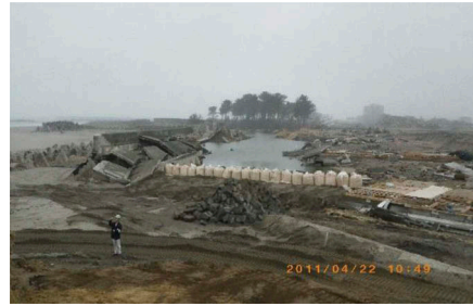
Figure 6. Damaged seawall near the Abukuma River mouth.
