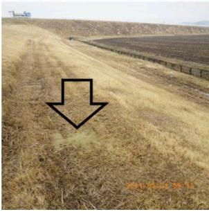
Figure 33. Sand ejecta from the middle height of a levee (Yoshida River, Miyagi Prefecture).
