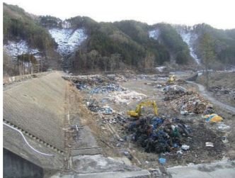
Figure 7. Destroyed community behind seawall (Tohni-Hongo).
